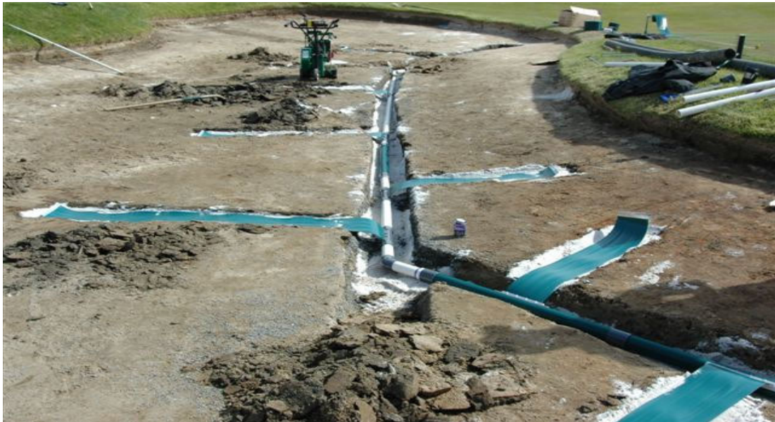
Figure 6 Smart Drain/Capiphon installed in a field ( http://www.smartdrain.com/ ).
