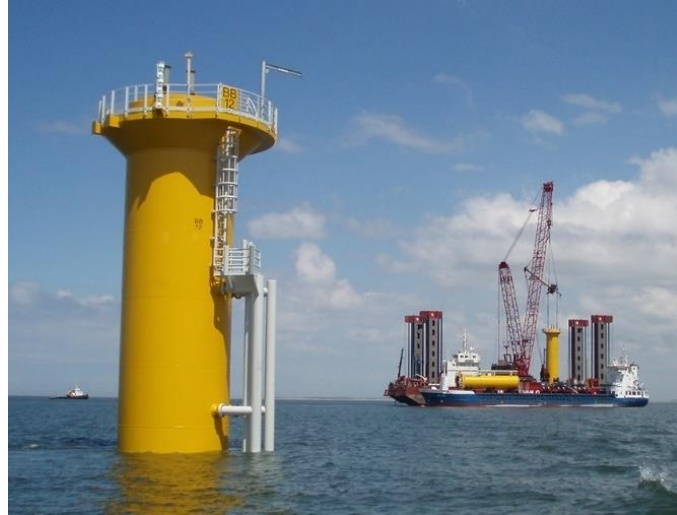
Figure 2.10: Installation of monopile transition piece with platform and appurtenances in Anholt, Denmark (Photo source: Ramboll, 2017)
