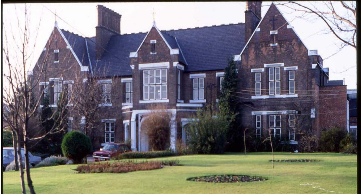
Figure 2: Entrance to Birmingham Workhouse. 2
