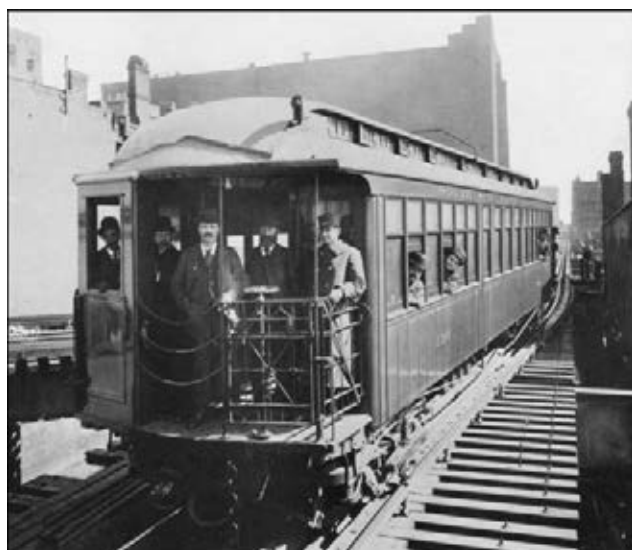
Figure 13: Chicago South Side Elevated car on a demo run in 1898. The driver's cab is the cubicle on the right. Sprague himself can be seen second from the left, standing in the back of the cab. The rest of the riders are company officials and their hangers-on. The general design of the car was to be adopted for the first electric fleets of most of the Underground lines in London. Photo: CERA.
