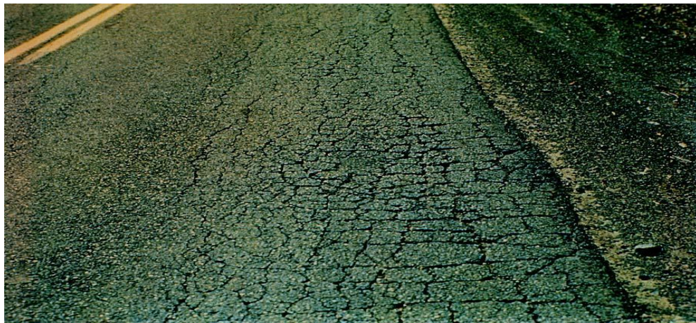
Figure 2. 7 Fatigue cracking (PavementInteractive, 7 April 2009)
