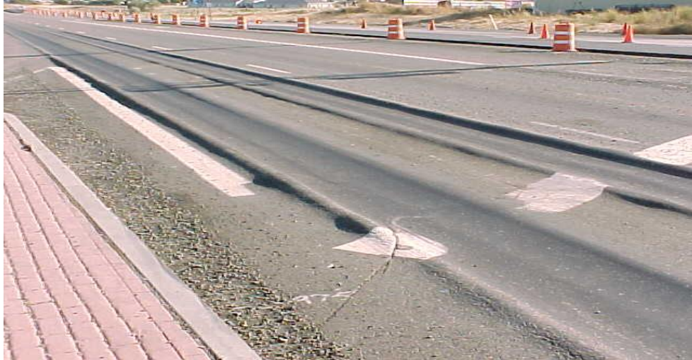
Figure 2. 8 Rutting (PavementInteractive, 6 May 2008)
