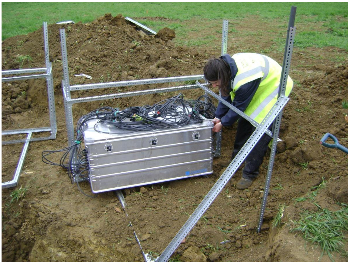
Figure 3.19: The construction of the solar panel mounting frame and positioning of the monitoring stations
