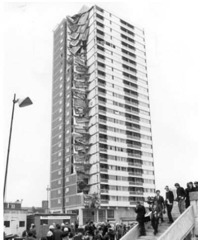
Figure 2.6 Ronan Point building progressive collapse -16 May 1968 (Nair, 2005)
