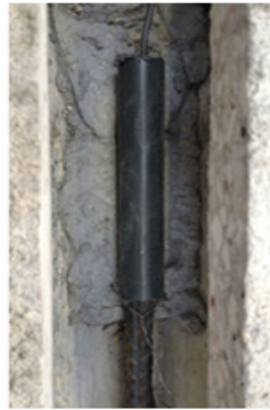
Figure 3.22 Plastic tube at the bar end
