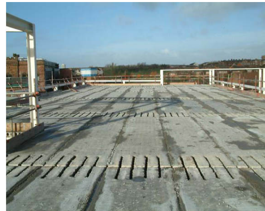
(b) Examples of longitudinal ties (Courtesy of Bison Concrete)
