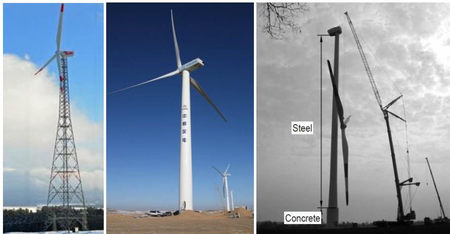
a. Lattice tower (Knight, 2014) b. Tubular tower (Wikipedia, 2014b) c. Hybrid tower (Gasch and Tvele, 2012)
