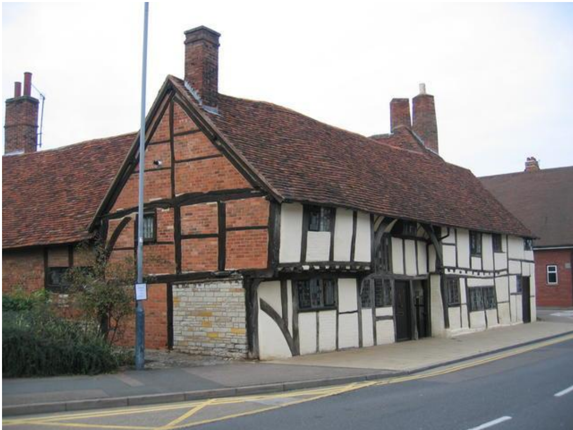
Figure 11 Mason's Court on Rother Street, Stratford-upon-Avon. 'Wealden' house type, dating to 1450, with square framing c. 1600. Image © David Stowell
