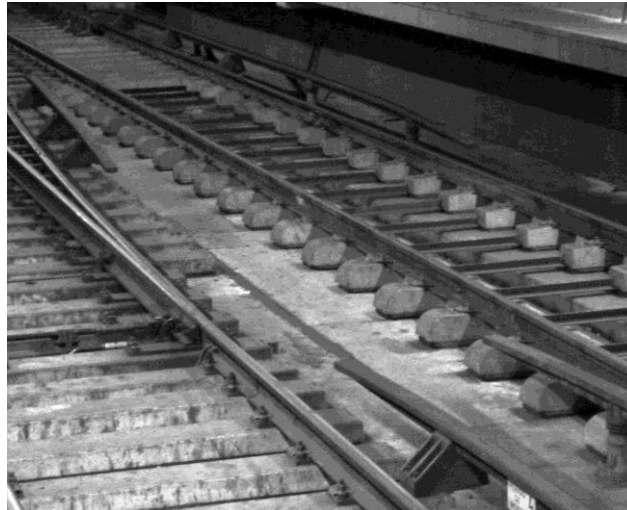
Figure 1: Gap in 3rd Rail Electrification Infrastructure (Hoffrichter 2011)
