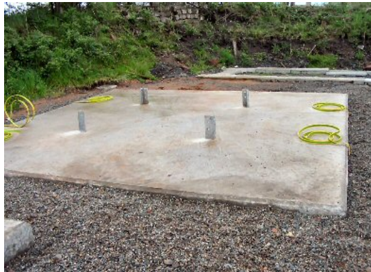
Figure 8.12: Typical mass concrete base
