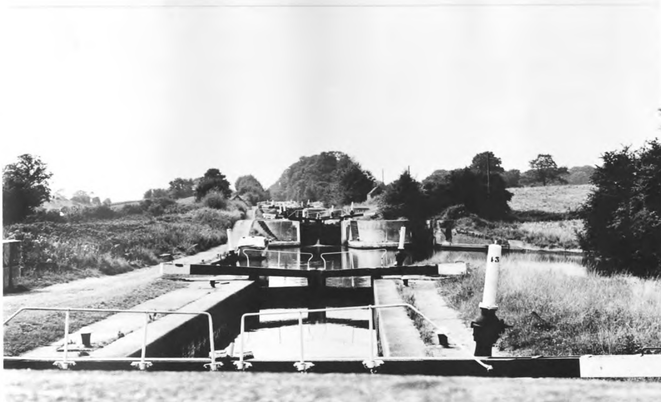
Plate 2: VIEW OF HATTON LOCKS LOOKING NORTH. The descent from the sharp edge of the Birmingham Plateau to the Avon Valley necessitated the construction of a flight of twenty-one locks.
