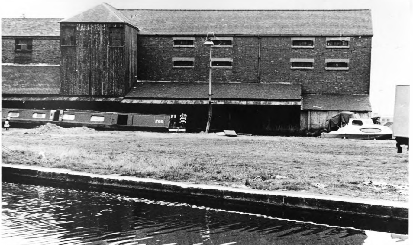
Plate 12: THE COVENTRY CANAL COMPANY'S WAREHOUSE AT LEICESTER ROW BASIN, COVENTRY. The small regular windows at a high level guarded unauthorized entry.
