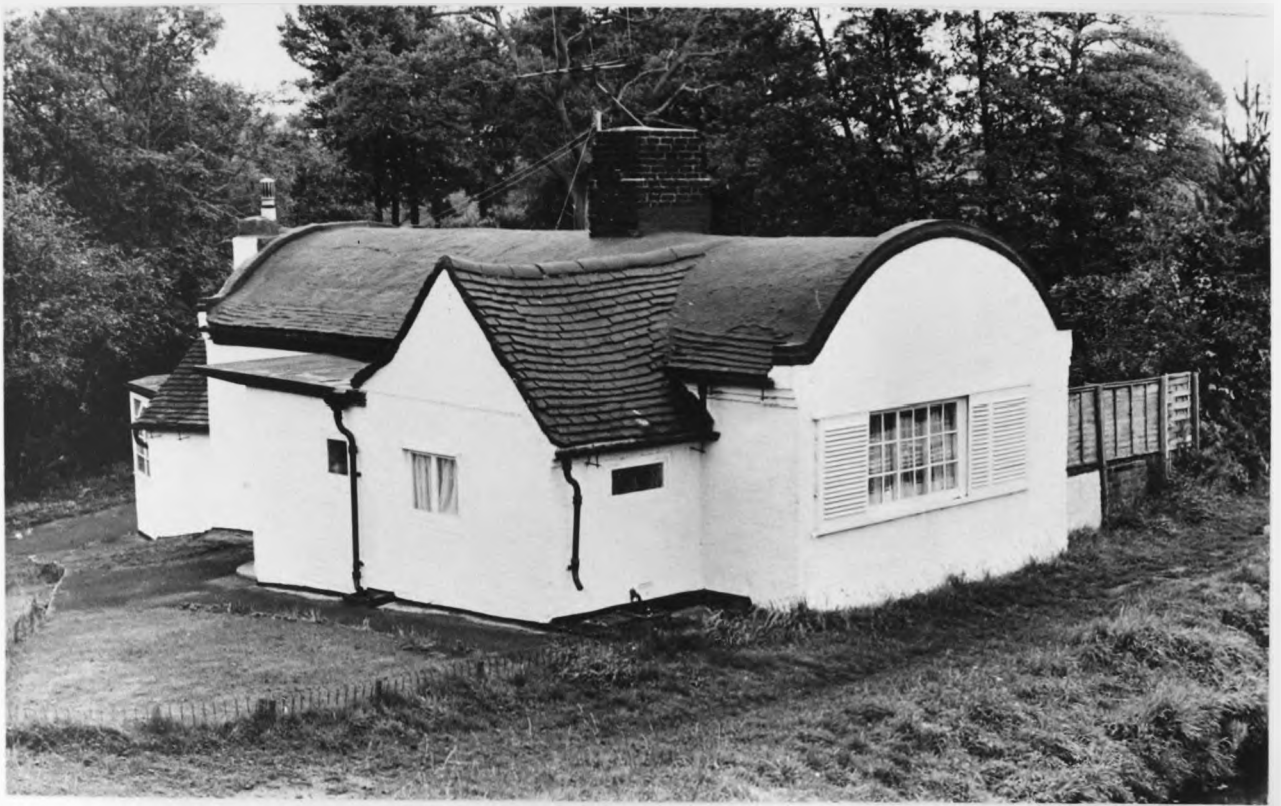
Plate 20: A BARREL-VAULTED ROOF COTTAGE AT DICKEN'S LANE. (Stratford-upon-Avon Canal). This interesting architectural form was based on tunnel design and effectively combined durability with economy. The tiled section was added later.
