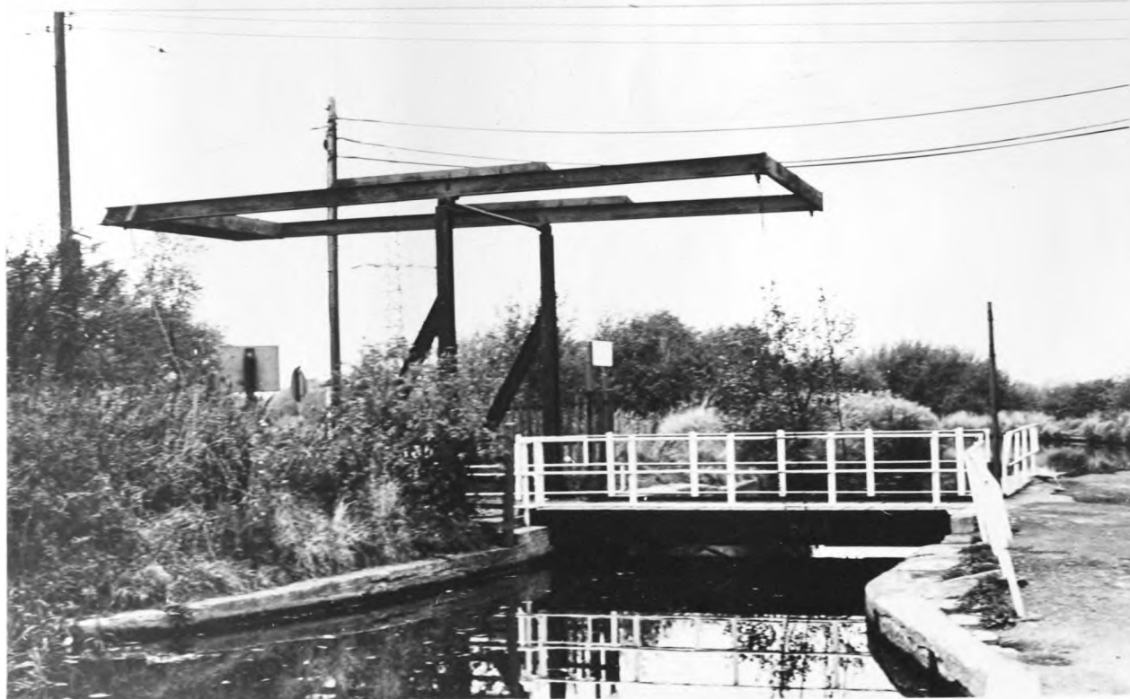
Plate 23: THE CANTILEVER BRIDGE AT SHIRLEY (STRATFORD CANAL). This was one of the cheapest types of canal bridges to construct.
