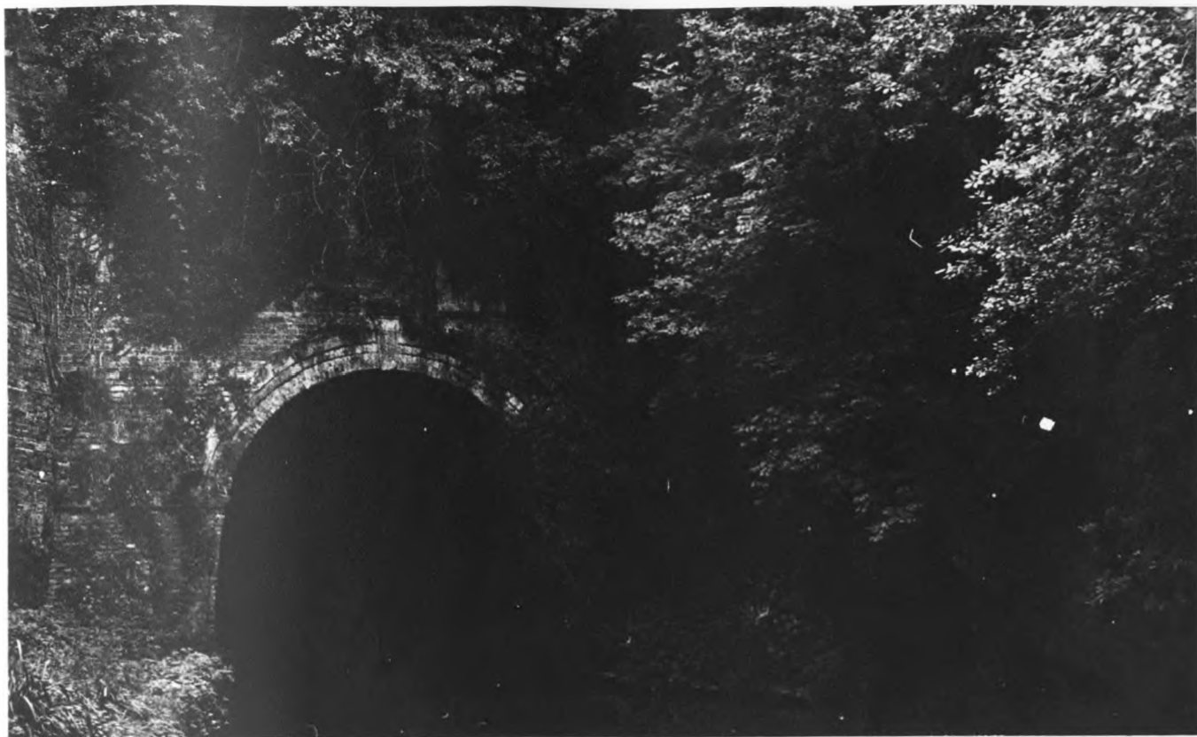
Plate 1: SOUTHERN ENTRANCE TO THE SHREWLEY TUNNEL. This tunnel, 433 yards long, cut through Keuper Marl, maintained the level of the Birmingham-Warwick Canal at 337' 5" from Knowle to Hatton.
