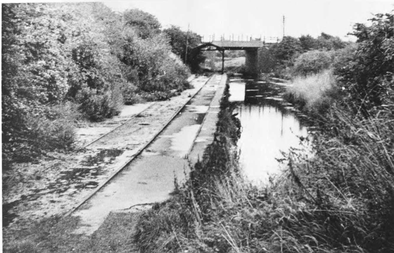
Plate 7: THE GRIFF HOLLOWS CANAL (1787) NEAR MARSTON JABBETT. This linked the Arbury coalfield to the Coventry Canal. Note the tramway which carried coal from the wharf.
