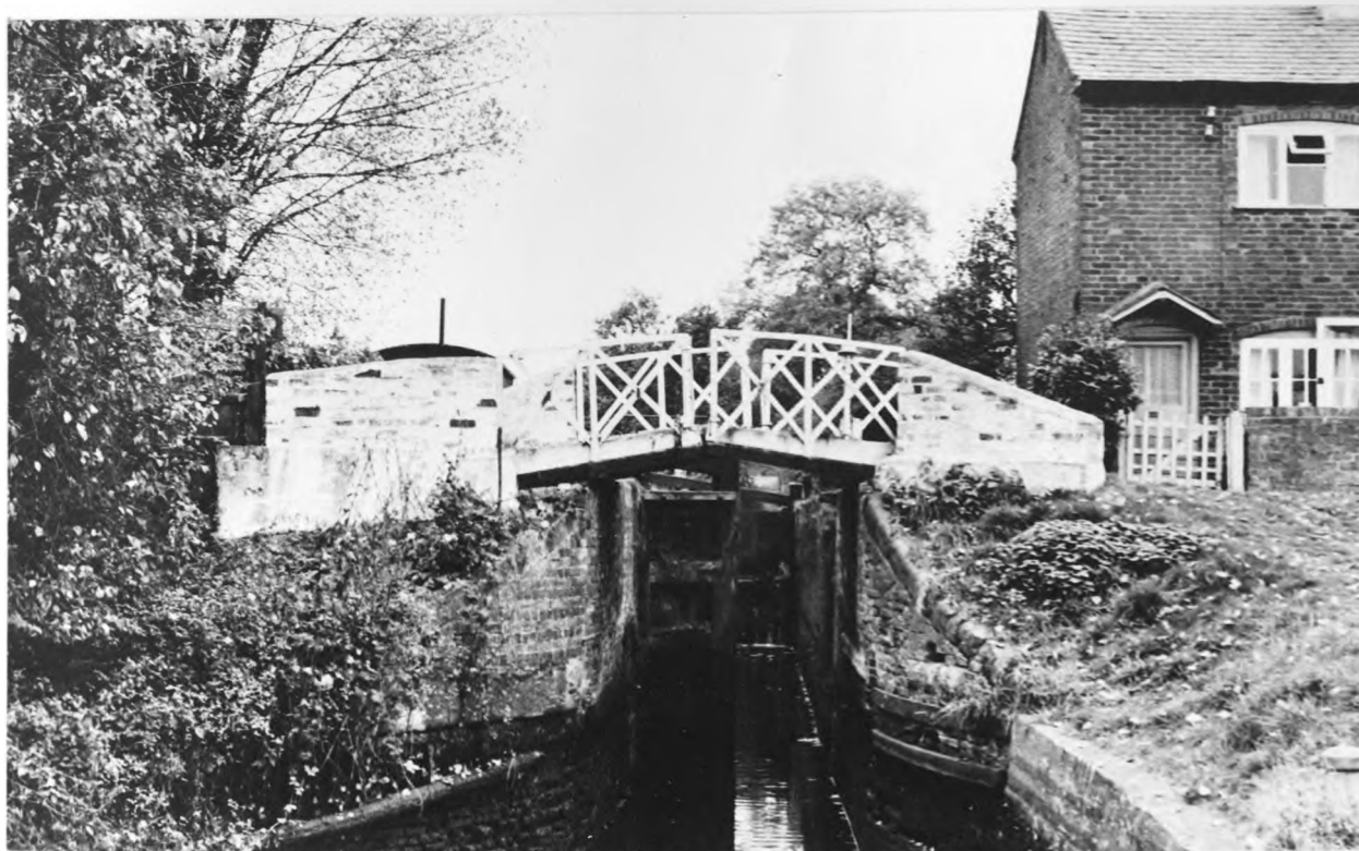
Plate 25: A CAST-IRON SPLIT BRIDGE AT LAPWORTH . This interesting construction had no towpath, but the slit allowed an easy passage of the tow-rope. The horse was led over the bridge. Lock-keepers cottage with modified windows on right.
