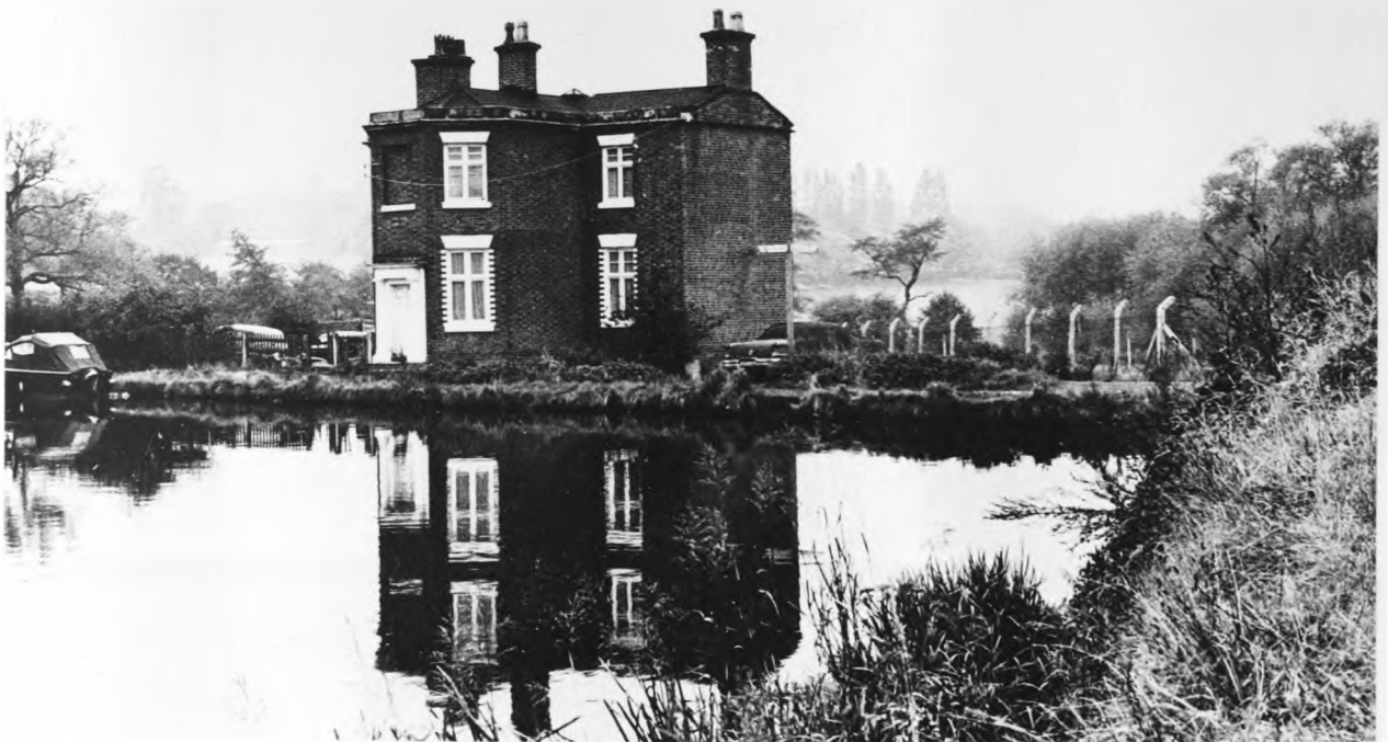
Plate 21: TOLL-KEEPER'S COTTAGE AT THE JUNCTION OF THE STRATFORD AND THE WORCESTER-BIRMINGHAM CANALS. A distinctive "canal style" is revealed in the gaunt brick cottages, slate roofs and long rectangular windows shown in Plates 19, 21, 22.
