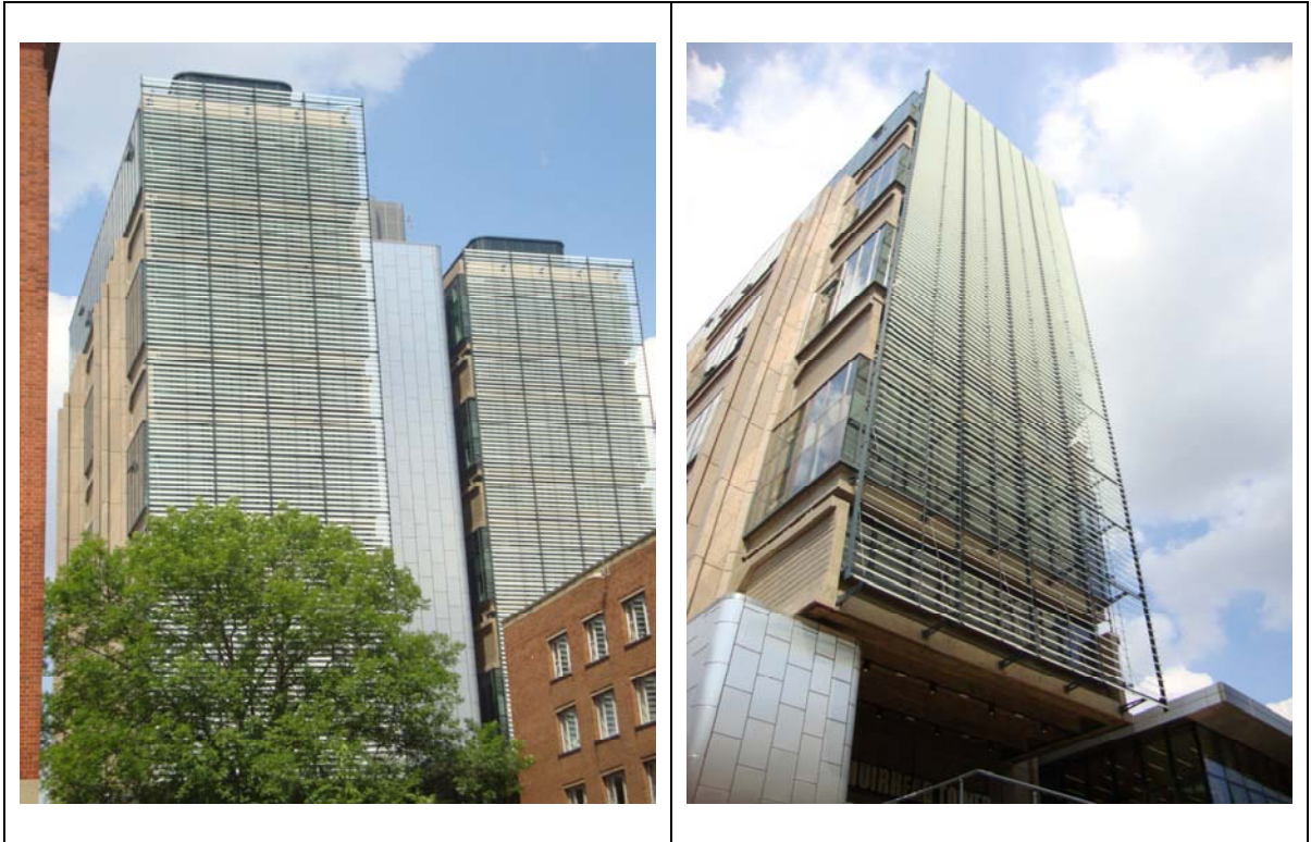
Figure 6.7 Using Koolshade system in Muirhead Tower
