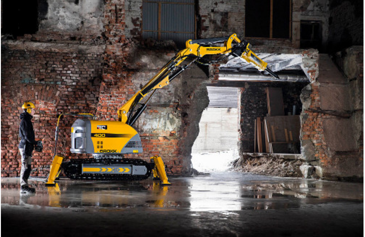
Figure 8.2: The Brook company is one of the leader in the field of robotic demolition. The picture shows a robot teleoperated by the human operator for dismantling an old building.
