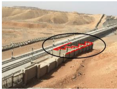
Figure 1.2: Part of the of Lanzhou–Xinjiang railway line, comprising of a transition region in the windbreak wall (Chen et al., 2021).
