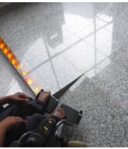
Figure 6-12 Change of floor level (a) a caution sticker is placed to warn user of the level changes (b) separate route for wheelchair is provided
