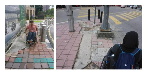
Figure 6-40 Poorly repaired/reinstallation of pavement surface
