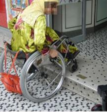
Figure 6-5 Examples of shop lot entrances (a) a gentle slope replacing raised/dropped floor (b) shop entrance with raised floor
