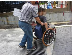
Figure 6-54 Grating drain cover (a) big gap in between two piece of gratings (b) participant was not confident to wheel through the grating vertically
