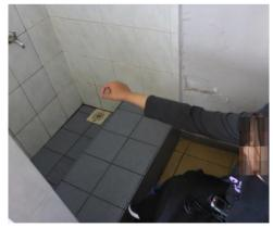
Figure 6-32 Examples of design of ablution area with kerbs that create barrier to user
