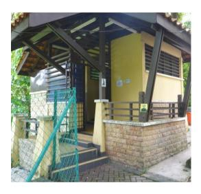
Figure 6-6 Inaccessible entrance for wheelchair to access surau
