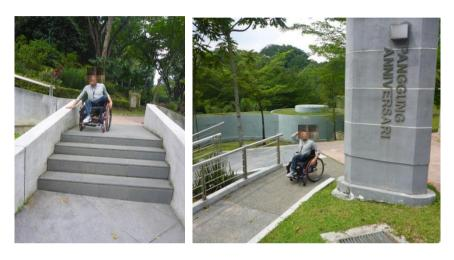
Figure 6-47 Access in a park (a) inaccessible steps (b) accessible ramp
