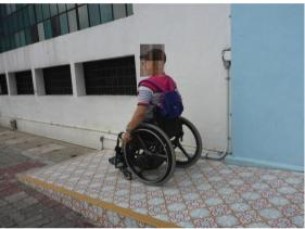
Figure 6-3 OKU access at Central Market main entrance (a) a ramp is provided adjacent to the steps (b) the ramp is lacking in user safety precaution
