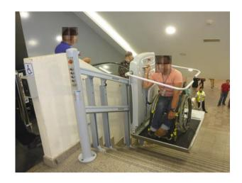
Figure 5-6 Stair lift provided to access Suria KLCC from the KLCC Station (subway)
