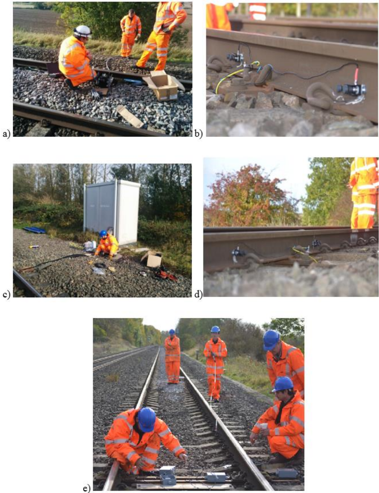
Figure 47: Photographs showing the installation of the customised 12-channel AE-vibration system at the Cropredy site, direction from London towards Birmingham.
