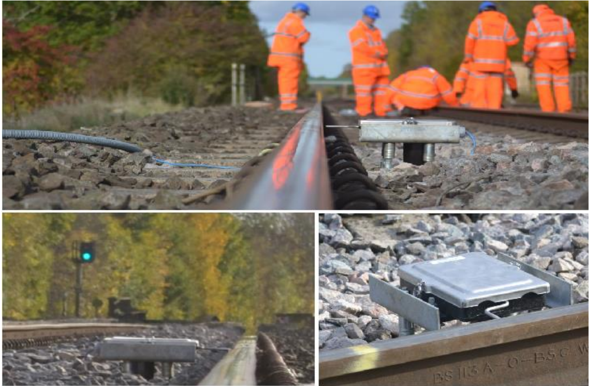
Figure 30 : A Treadle system installed on the Chiltern rail line between Banbury and Leamington Spa station.
