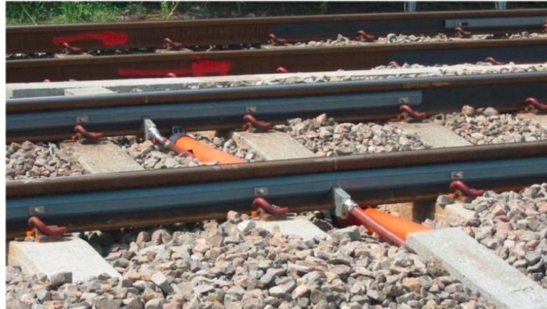
Figure 28: Photograph of a Wheelcheck system (the photograph is courtesy of Network Rail).
