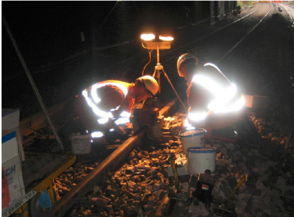
Figure 24: Aluminothermic weld preparation, Shugborough Tunnel, December 2012.
