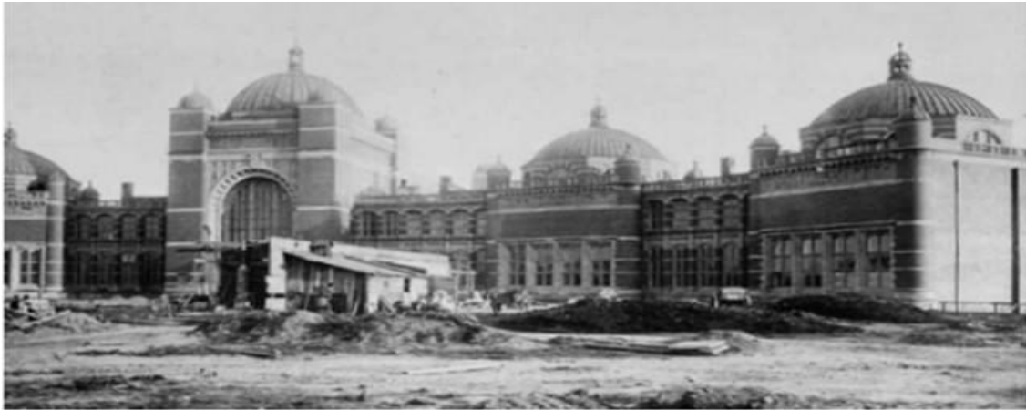
Figure 5.2. The University under construction in 1902 (University of Birmingham, 2012).
