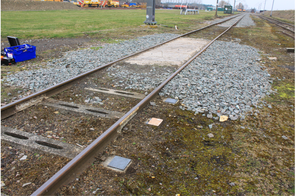
Figure 7.8: An overview photograph of the instrumented track
