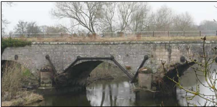
Figure 45 Vyrnwy Aqueduct, built by Hazledine and Simpson in 1797, and strengthened with wrought-iron rods and tie bars supplied by Hazledine in 1823 (the author)
