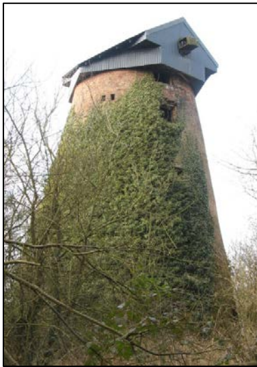
Figure 25 Remains of Hawkstone Mill. Notice the massive cast-iron canister which pierces the temporary cap (the author)
