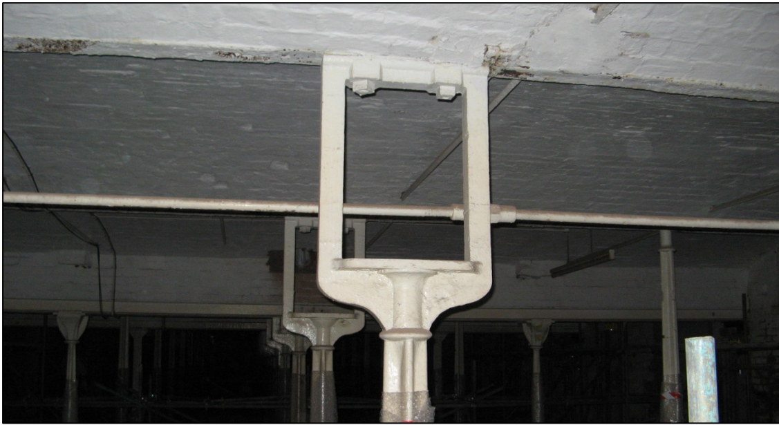
Figure 42 shows how the capitals of the central columns on the ground floor are cast to allow drive shafts for machinery to pass through and along the building. Note also the brick jack-arch floor above and the wrought-iron tie rod (the author)
