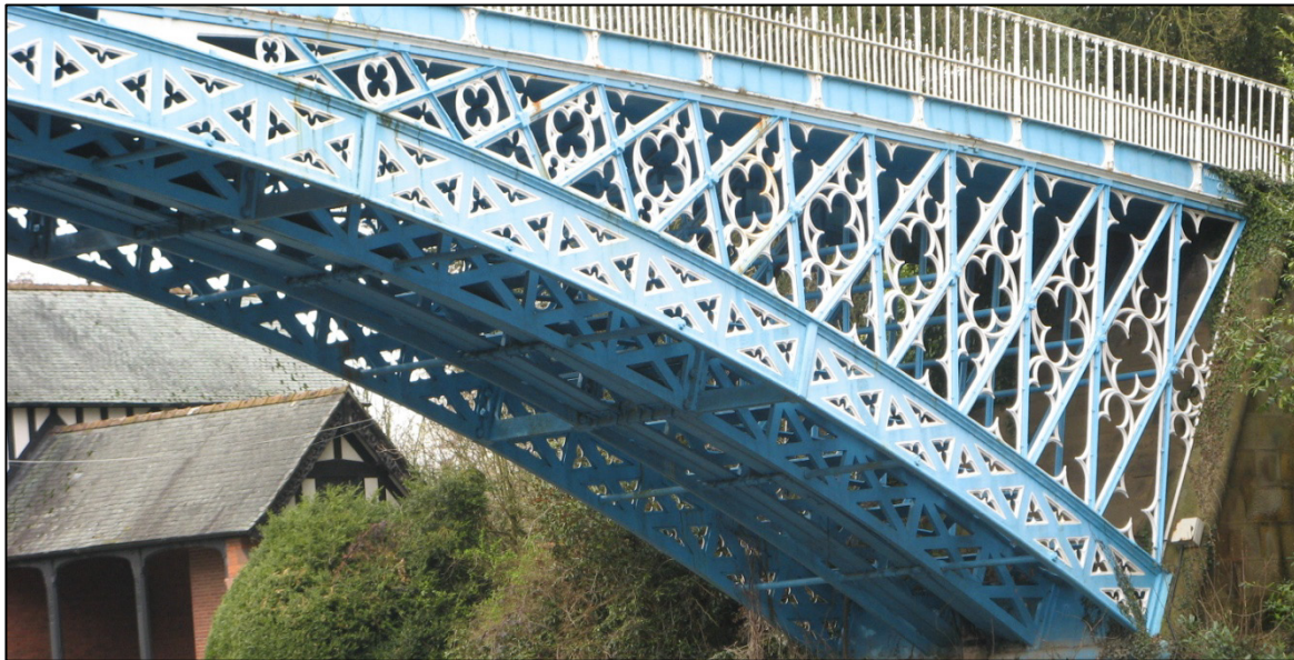
Figure 78 Eaton Hall Bridge – detail of decorative spandrel bracings. Notice trademark 'Hazledine' railings (the author)
