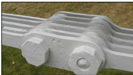
Figure 59 – Conwy Bridge - showing two sets of six flat-plate eye-bars joined by six connecting plates
