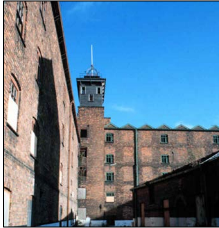
Figure 39 Ditherington Flax Mill, general view. Notice the 'saw-tooth' roof profile. Many of the original windows are now bricked up (the author)
