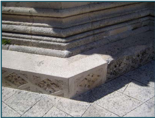
Fig 31. Reconstructed stonework on the South base (Clancy 2008)
