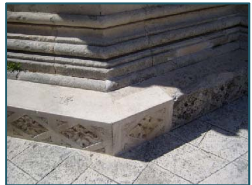
Fig 31. Reconstruction of the South base of the cathedral (Clancy 2008)
