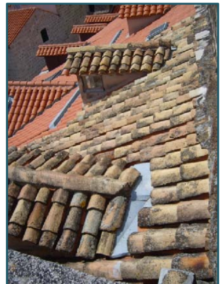
Fig 6. Old and new roof tiles, Dubrovnik (Clancy 2008)
