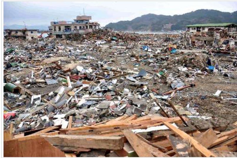
FIGURE 1.1 OTSUCHI TOWN (10 DAYS AFTER THE EARTHQUAKE AND TSUNAMI)
