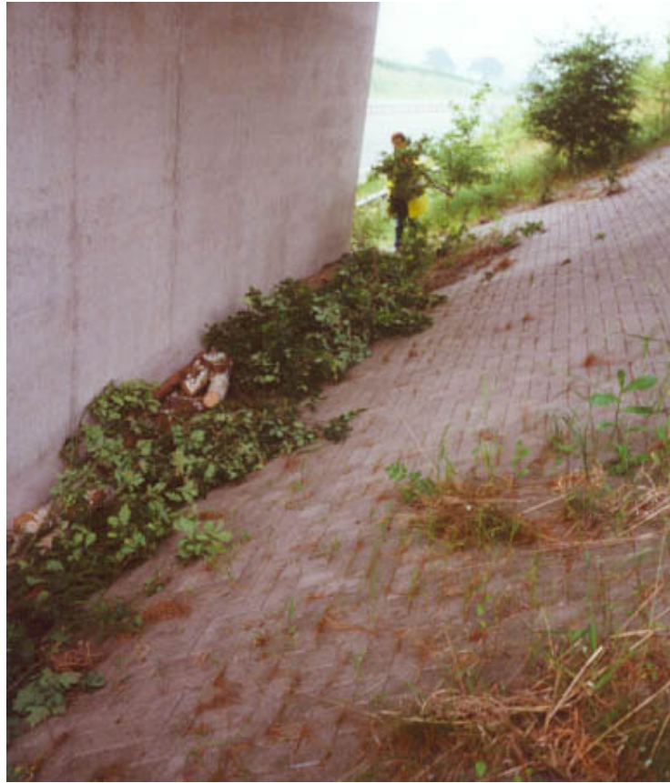
Figure 5.2 Installing cover beneath road bridges.
