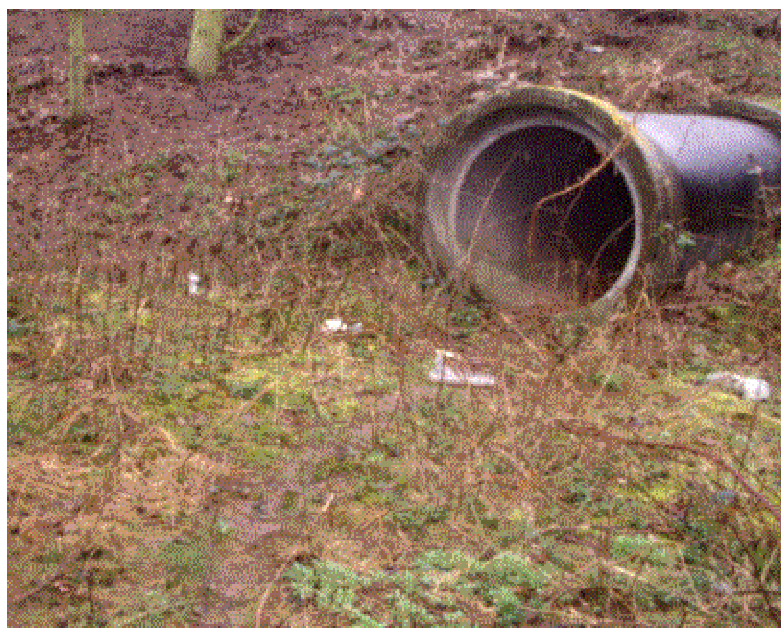
Figure 6.3 The entrance of one of the badger tunnels installed beneath the M40 motorway.
