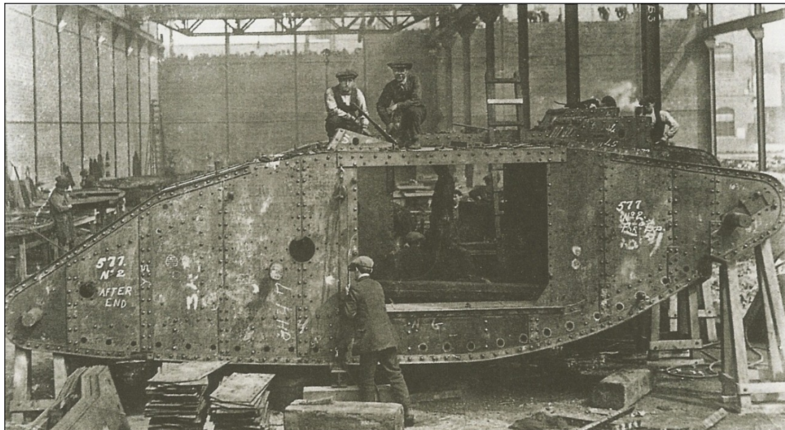
50. Mark II Tank under construction, winter 1916/1917. Source: K. Beddoes and C & S Wheeler, Metro-Cammell: 150 Years of Craftsmanship (Huddersfield: Runpast Publishing, 1999), p. 28.
