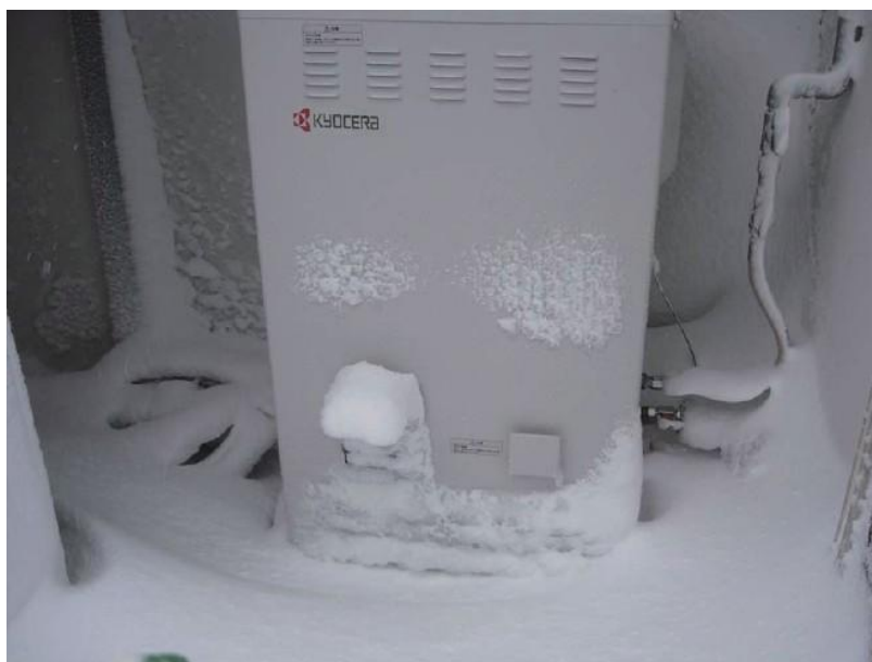
Figure 2.7: A Kyocera system installed in northern Japan, pictured operating at -17°C external temperature.
