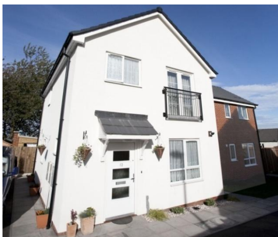
Figure 5.1: A photo of the 'hydrogen house' in the Black Country. The house was newly built in 2007 to above standard regulations, featuring double glazing and cavity wall insulation, with a floor area of approximately 100m 2 . [245]
