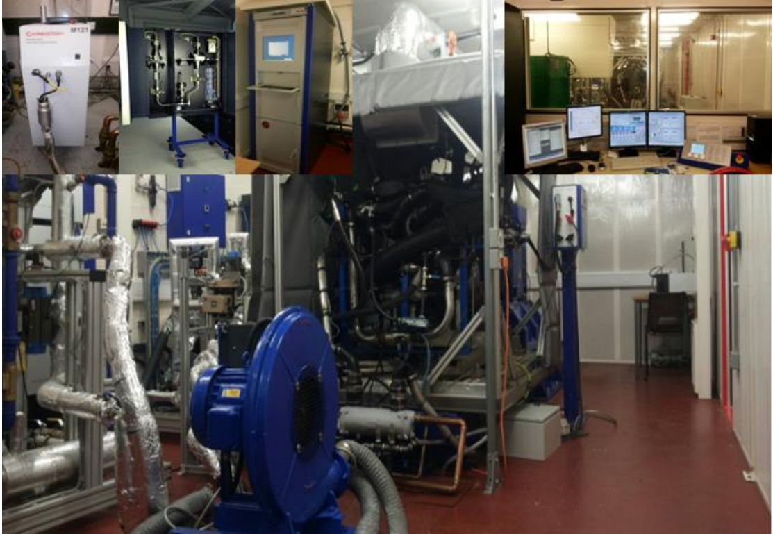
Figure 3.7 Test bench and facilities for climate change transient experiments
