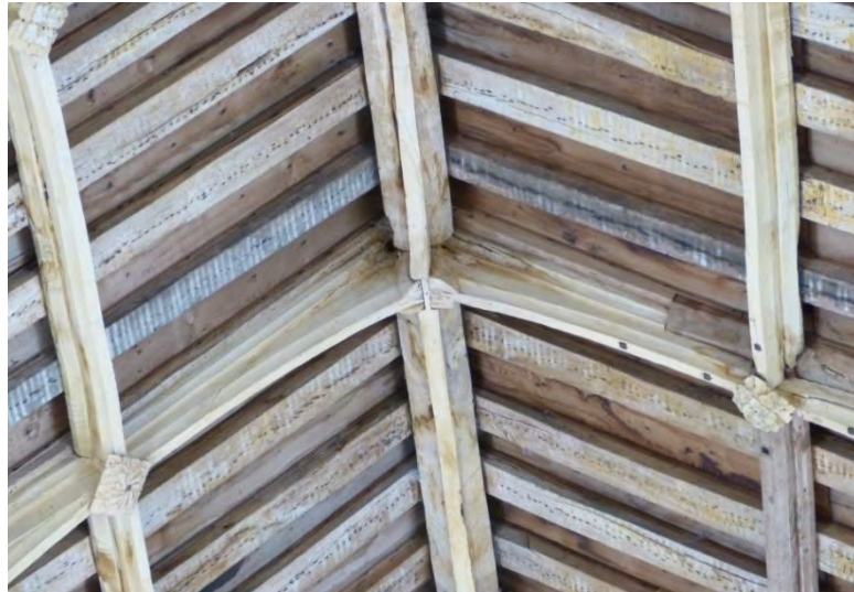
Fig. 8.16: Flared upper principals, Beeston-next-Mileham, Norfolk, nave roof.
