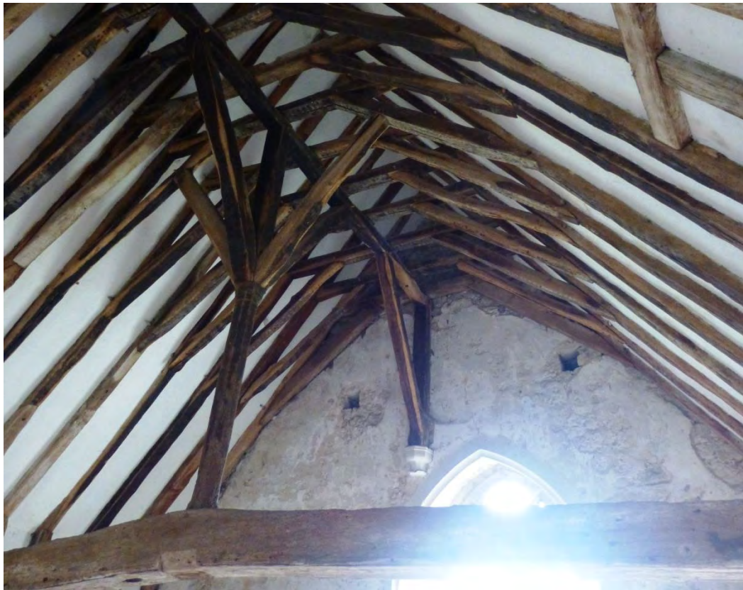
Fig. 4.11: Old Soar Manor, Plaxtol, Kent, corbelled wall post and strut in the solar, late thirteenth-century.
