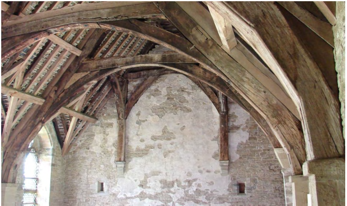
Fig. 4.9: Stokesay Castle, corbelled wall posts and struts against south gable.
