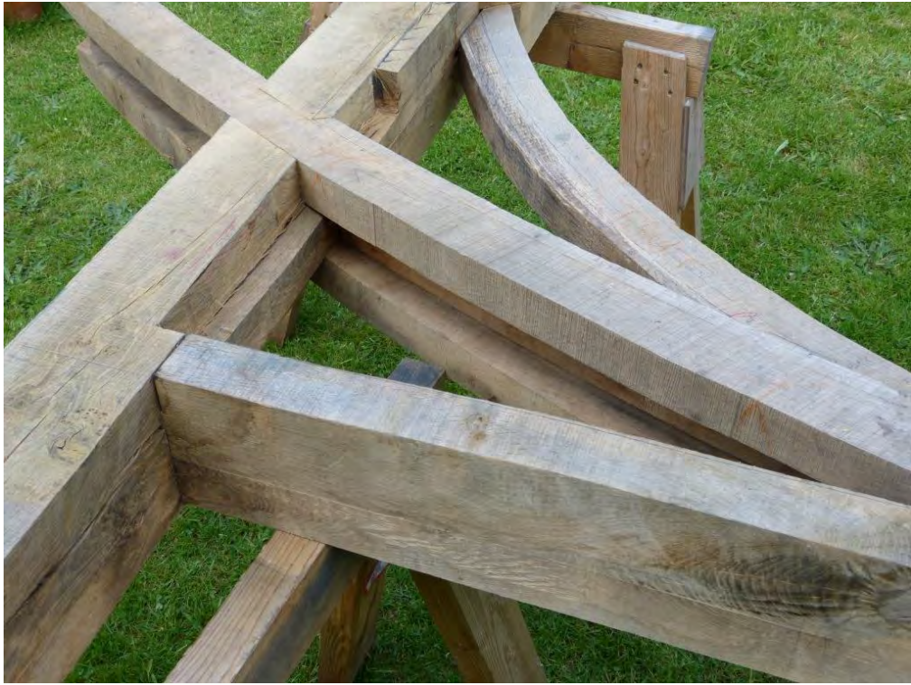
Fig. 6.20: Reconstruction of the Westminster Hall lower framing showing nature of arched rib before moulding; note u section formed by tripartite arched rib. The large timber running right to left in the foreground is the wall post.
