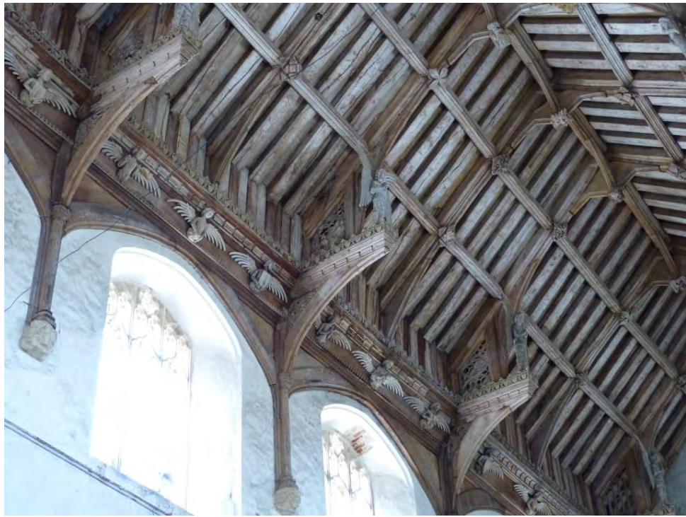
Fig. 3.25: Extended sole piece construction, nave of Cawston Church, Norfolk, mid C15. Ingression of the rafter foot is greater, facilitating a more elaborate cornice.
