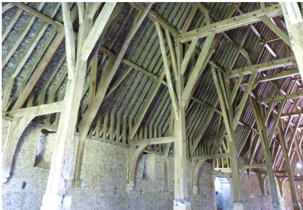
Fig. 4.14: Great Coxwell Barn, aisle-ties arch-braced to corbelled wall post, west wall.
