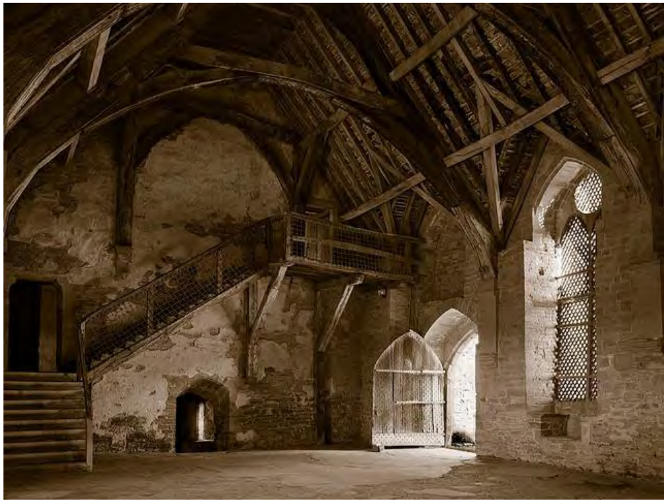
Fig. 3.27: Medieval bracketed structure: staircase, Great Hall, Stokesay Castle, c. 1290.
