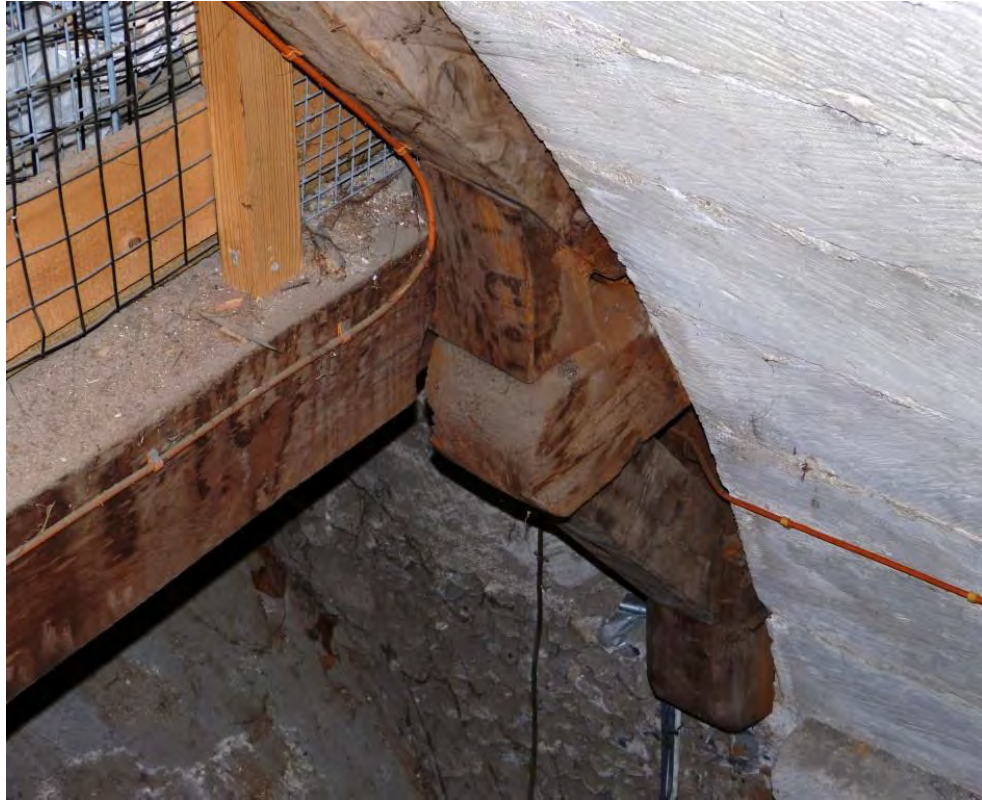
Fig. 4.19: Salisbury Cathedral, conjunction of north triforium and north porch roofs, detail of bracket. Walkway to left is a later insertion.
