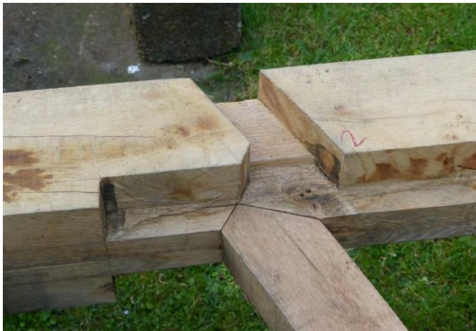
Fig 6.24: Reconstruction of Westminster framing, hammer beam / arched rib configuration; left: cogging of the hammer beam, note also the core is tenoned into the hammer beam; right, the outer laminate of the arched rib; note reduced section where it passes through the hammer beam.
