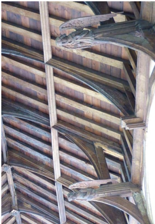
Fig. 8.44: Holme Hale Church Norfolk, nave, detail of roof-framing, fifteenth-century.
