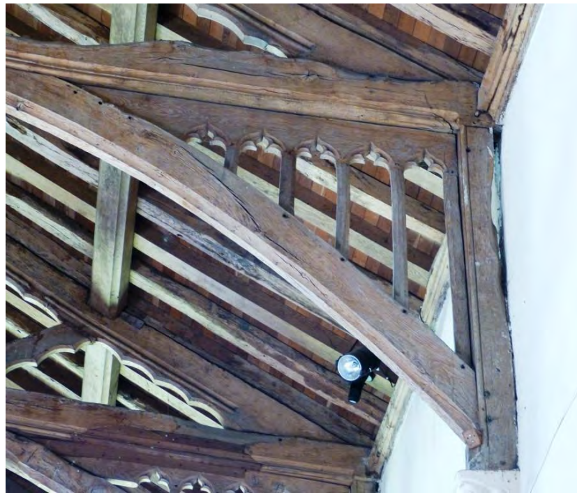
Fig. 6.5: Stanton Harcourt Church, Oxfordshire, detail of nave roof, c. 1400. Note how the arch brace is tenoned into the wall post horizontally, as evidenced by the vertical shoulder of the joint and the position of the pegs.
