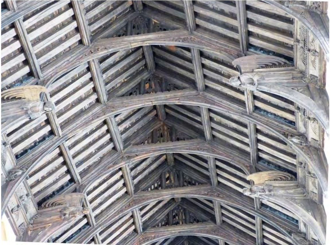
Fig 8.26: St Mary's, Bury St Edmunds, nave roof, detail of apex framing.
