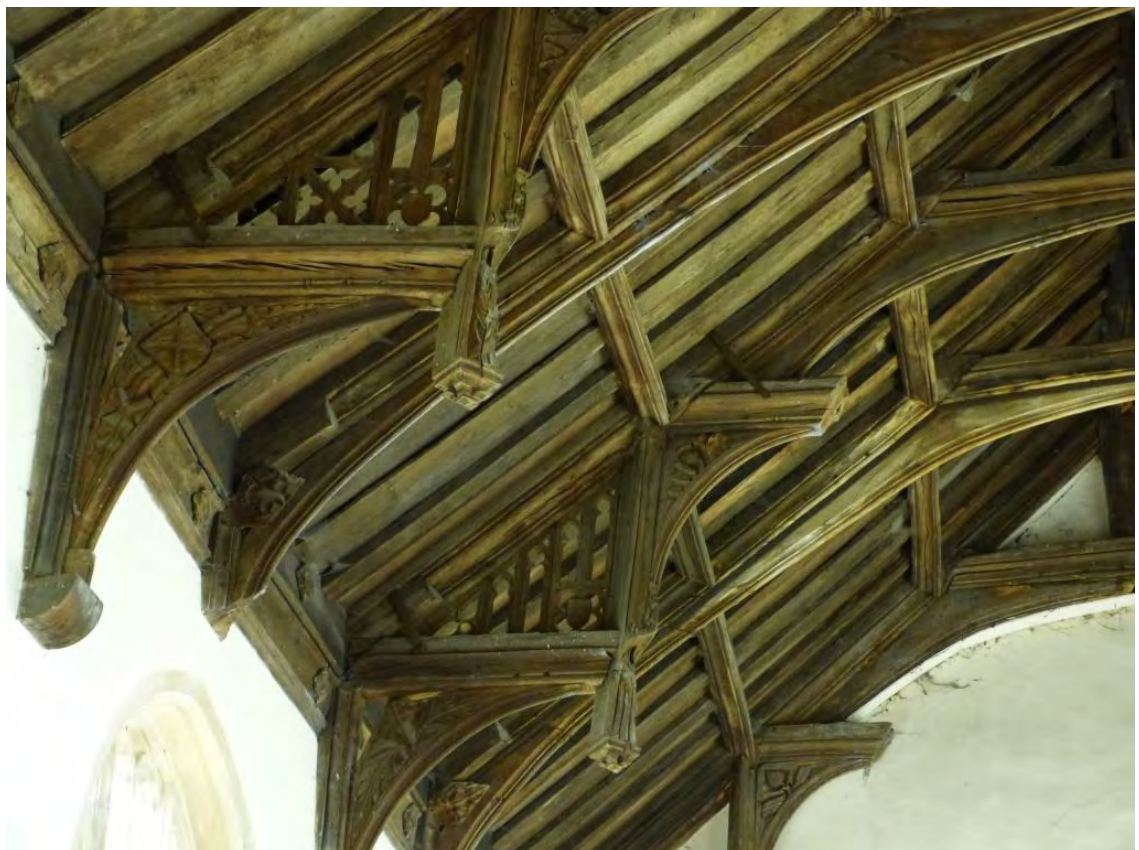
Fig. 8.36: Tostock Church, nave roof, detail of pendant post framing.
