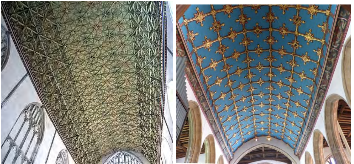
Fig. 1.35: Waggon roofs. Left: Canterbury Cathedral, Chapter House, 1397; right: St Mary's, Bury St Edmunds, chancel, fourteenth-century (restored C19). Note how the construction permits the horizontal termination of the wall head.
