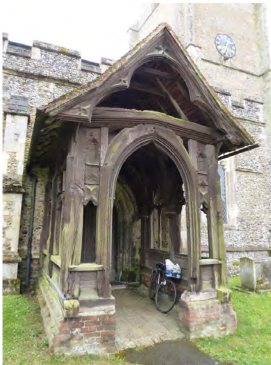
Fig. 6.6: Boxford Church, Suffolk, timber north porch, fourteenth-century; right: detail of wall post to rib framing.
