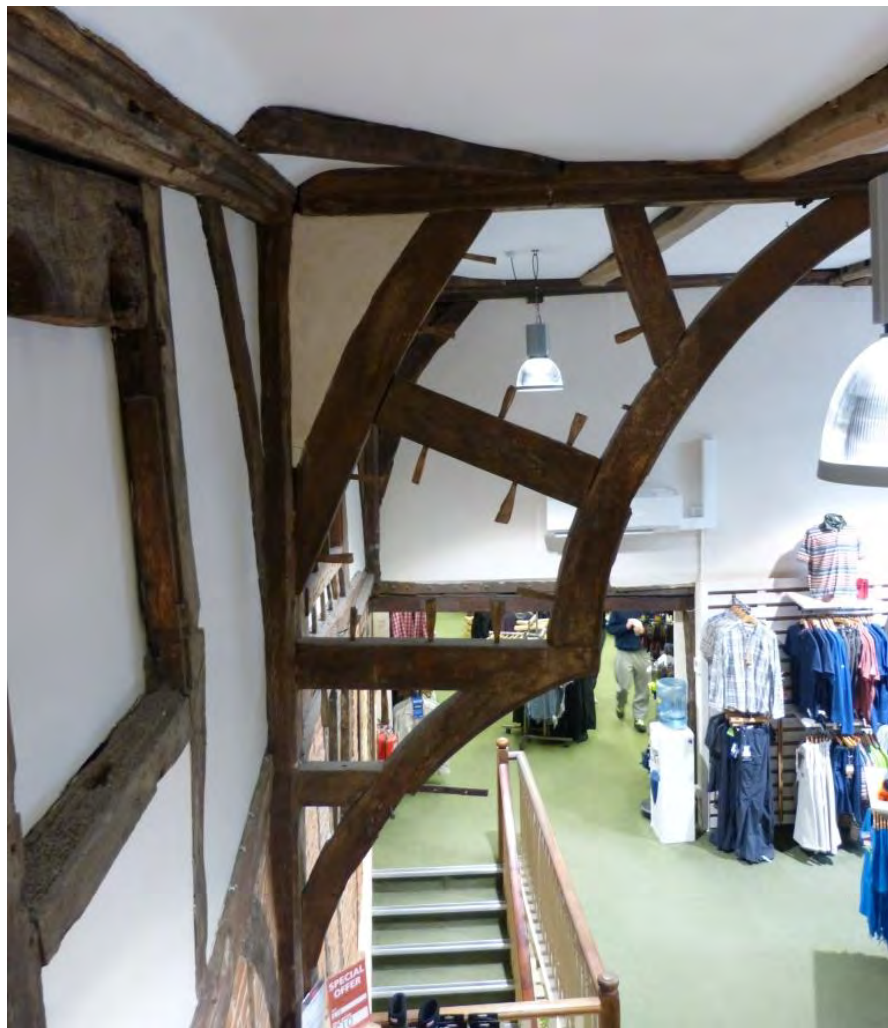
Fig. 4.42: William Russell's House, detail of tie-beam bracing. Note slight scanting in comparison to structural hammer-beam framing of the Pilgrims' Hall (Fig. 3.16)
