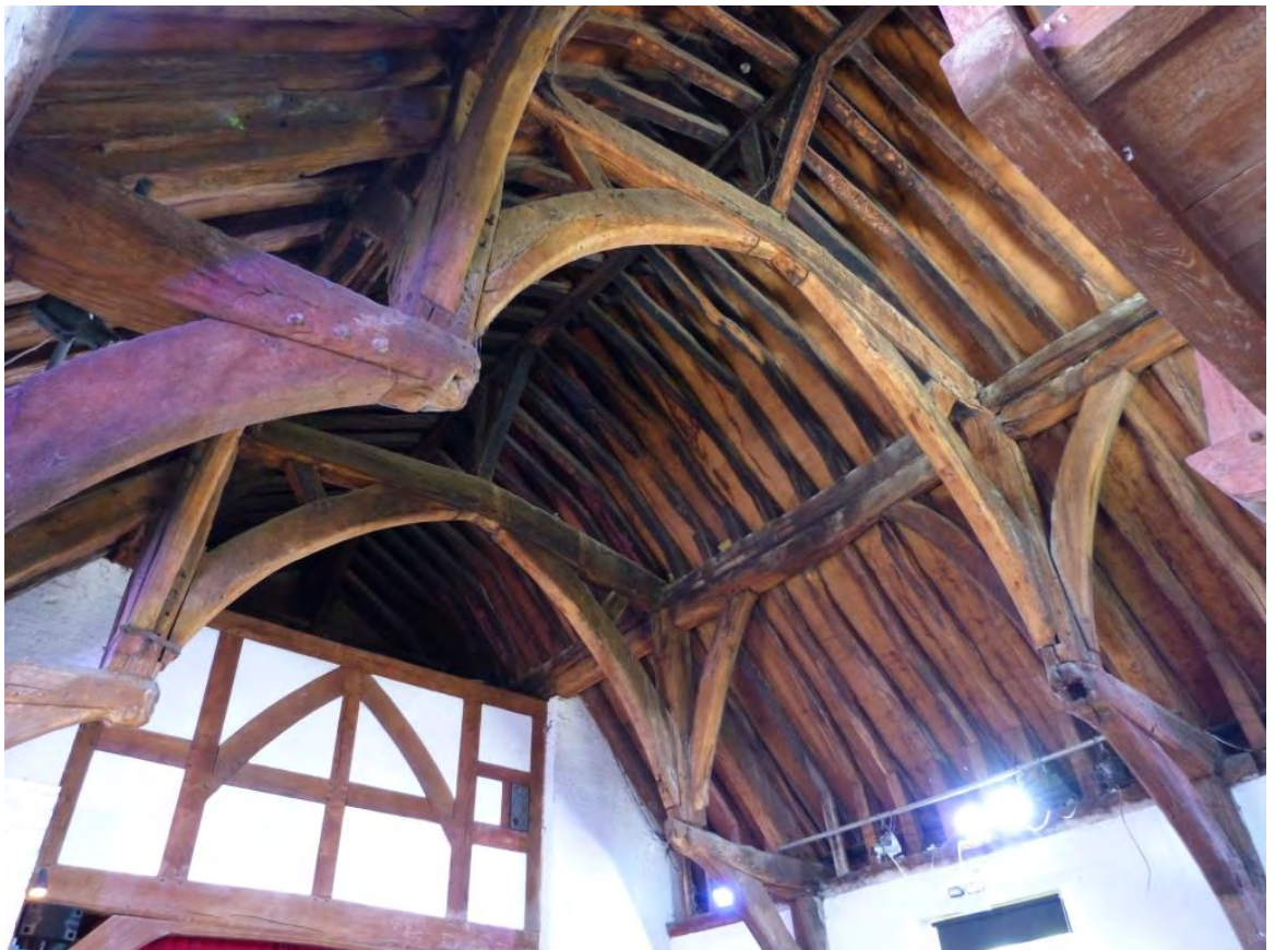
Fig. 3.16: Pilgrims' Hall. Note longitudinal bracing from base of hammer post to arcade plate, a configuration typical of aisled construction.
