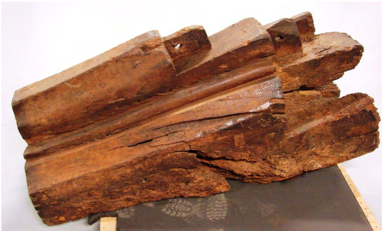
Fig. 6.27: Part of an original wall post from Westminster Hall removed during the restoration of 1914. Note, middle right, the lack of a tenon for the outer laminate, and the peg-hole (now split) showing how the laminate was simply face-pegged to the wall post. (Museum of London)
