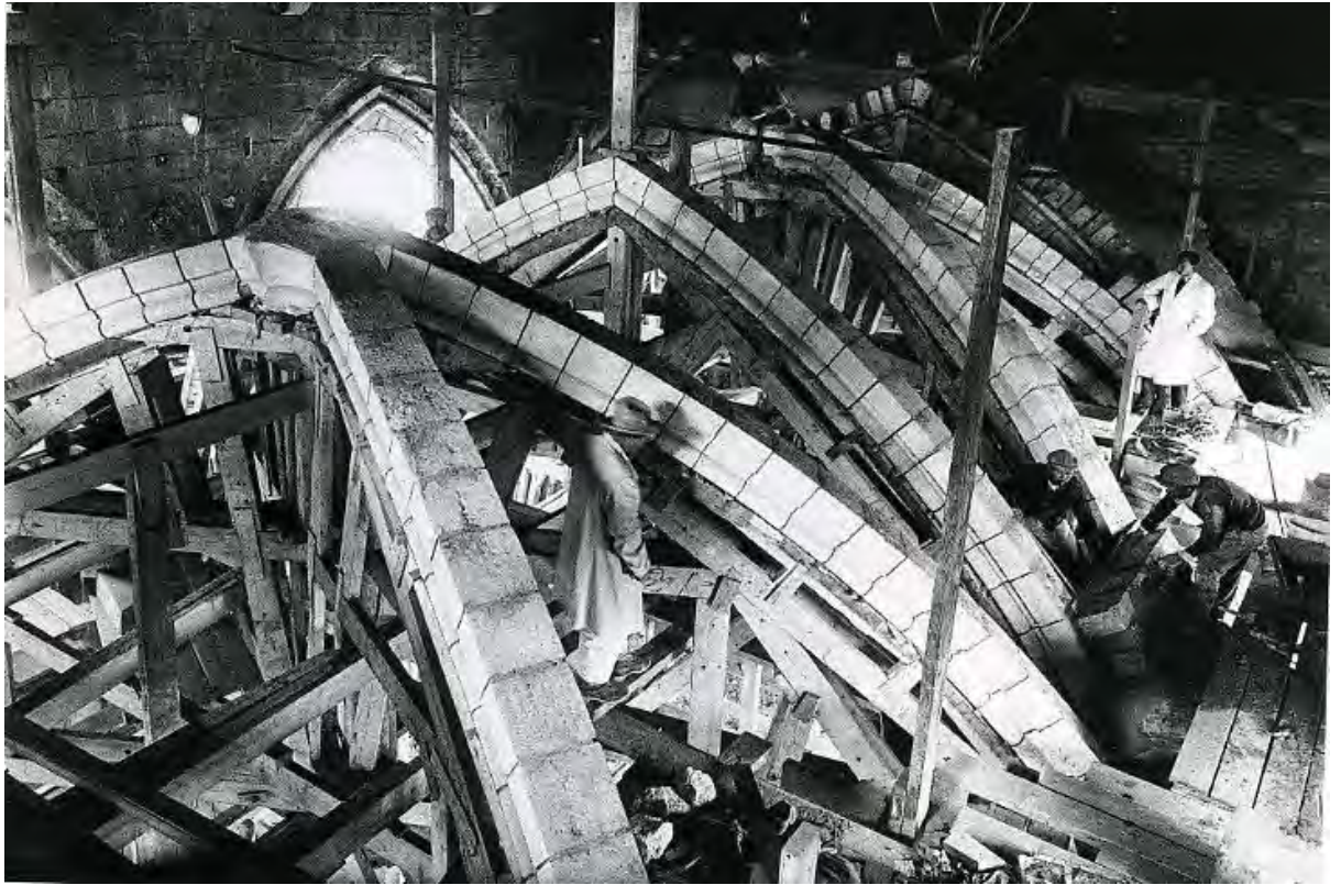
Fig. 1.19: Soissons Cathedral, nave vault under reconstruction following World War I.
