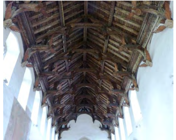
Fig. 1.47: Pendant post hammer-beam roofs. Clockwise from top left: Cotton Church Suffolk, c. 1471 (with alternate arch-braced frames); Wetherden, Suffolk; Grundisburgh; Suffolk (pendants are in the upper tier of hammer posts), both probably late fifteenth-century. Gestingthorpe Church, Essex, 1489. All double hammer-beams.
