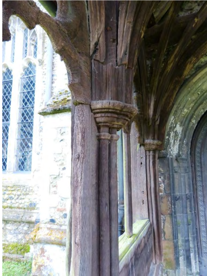
Fig.4.39: Boxford Church, north porch, detail of shafts and 'vault' springing.
