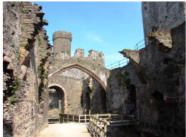
Fig. 7.4: Conway Castle, North Wales, great hall c. 1346, remains of roof. Left: mid-19 th century watercolour by J. H. Pollen. By the 20 th century only one arch remained, but note the springing points of the lost arches.
