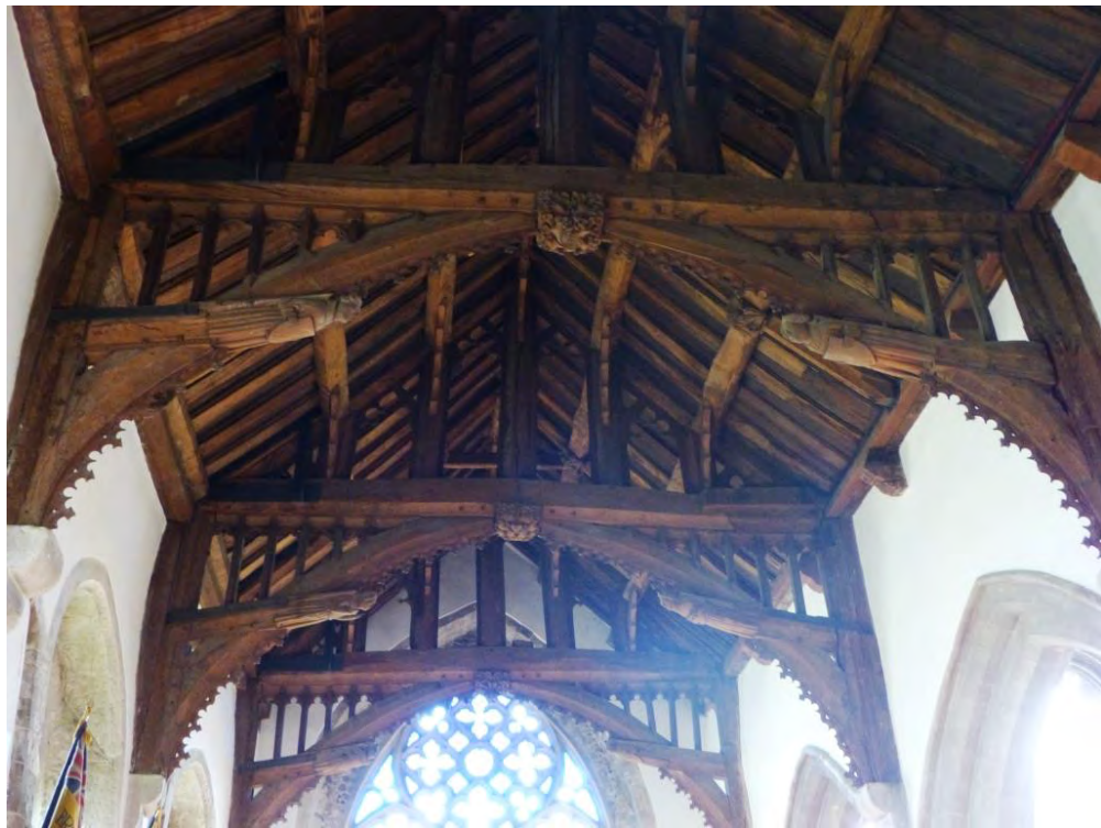
Fig. 4.34: Fordingbridge Church, Hampshire, north chapel, fifteenth-century. Angel 'hammer beams' interrupt arch braces to the tie beam.
