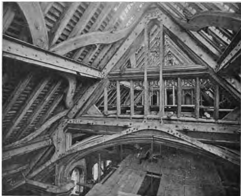
Fig. 8.50: Eltham Palace. Photograph taken during restoration in the early C20. Note the huge amount of riveted steelwork introduced to maintain the roof's structural integrity, (from Cescinsky & Gribble)
