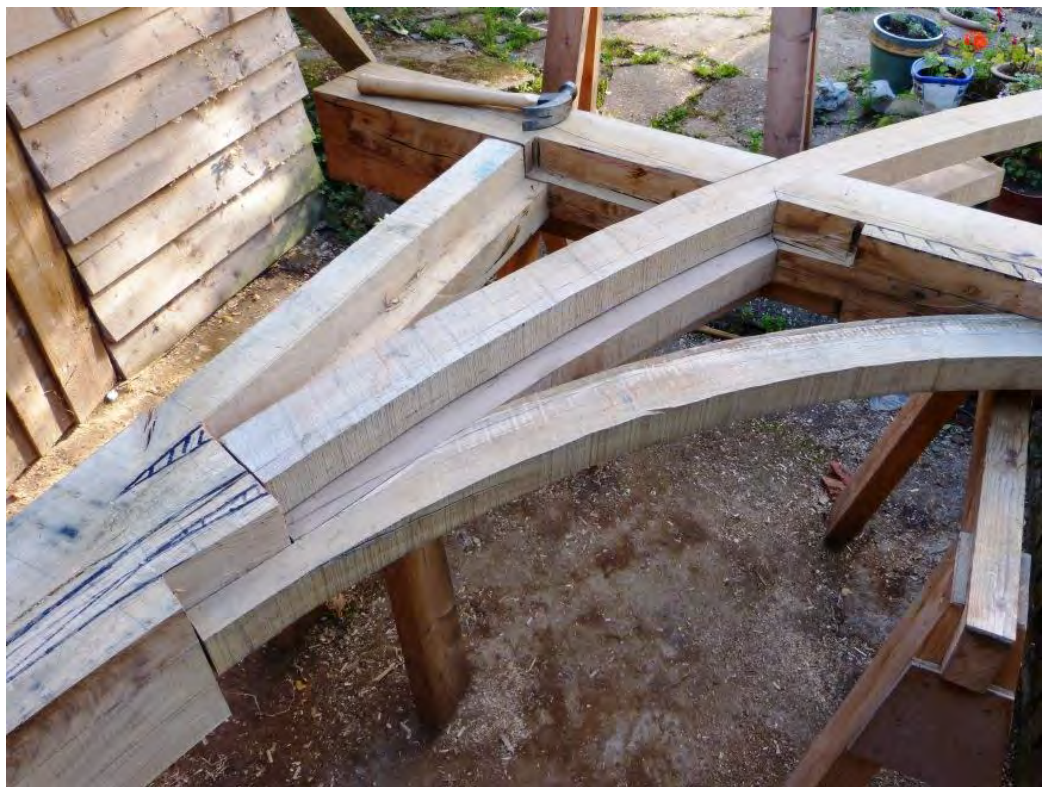
Fig. 6.31: Reconstruction of Westminster Hall framing, showing the complex contignation where the ribs meet the wall post.
