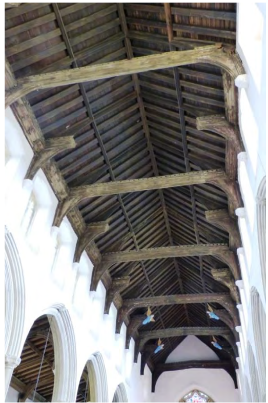
Fig. 8.7: Type 1.2 tie-beam / hammer-beam roofs. Left: Debenham Church, Suffolk, 1403 \pm 6d; right: Bildeston Church, Suffolk, c. 1420.
