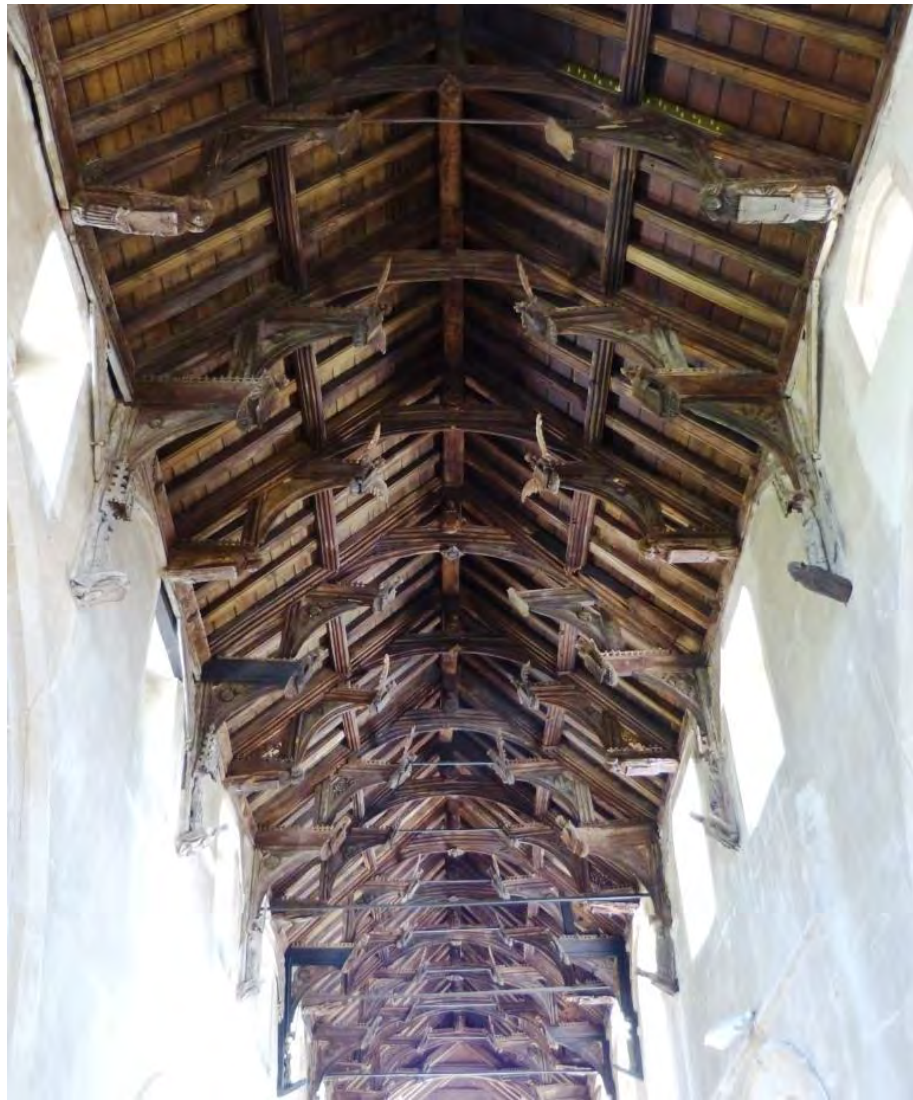
Fig. 8.1: Tilney All Saints Church, Norfolk; nave, double hammer-beam roof; probably 3 rd quarter of the fifteenth century.
