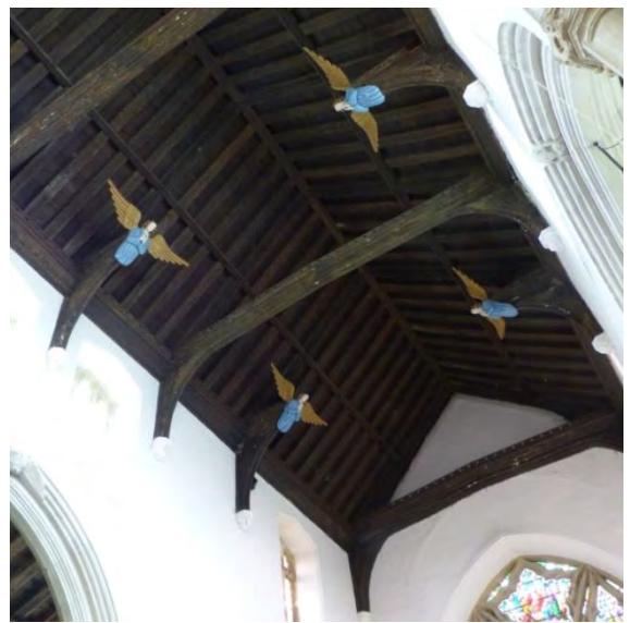
Fig. 8.8: Left: Debenham Church, note extant tenons on ends of hammer beams; right: Bildeston Church, replaced hammer-beam angels.
