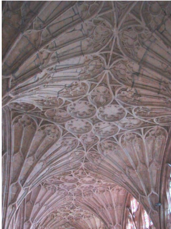
Fig. 1.39: The earliest English fan vault: Gloucester Cathedral, cloister, east walk, c. 1351-64, looking south.
