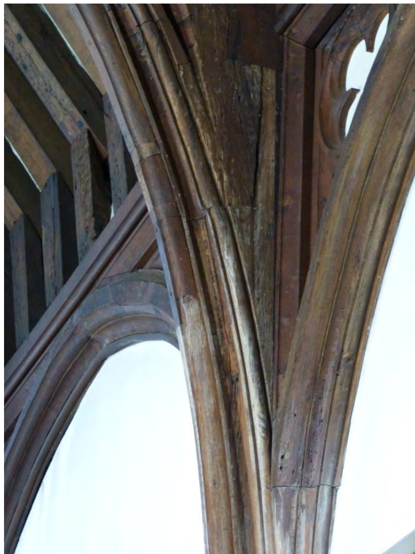
Fig. 7.18: The Guard Room, detail of framing at the springing of the arch rib and wall arcading.
