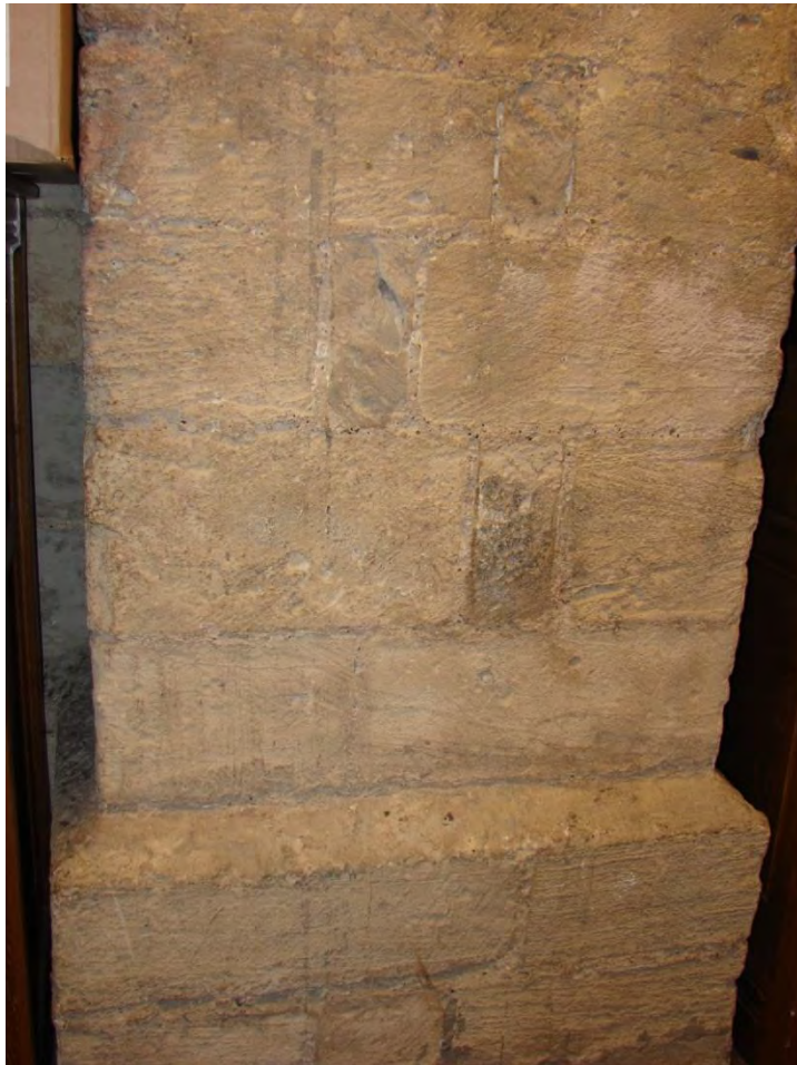
Figs 5.2 & 5.3: Westminster Hall, remains of Norman masonry in the lower portions of the west wall.
