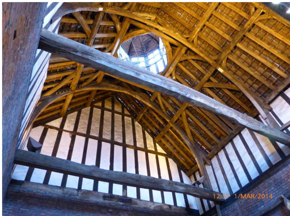
Fig. 4.26: Gainsborough Old Hall, Lincolnshire, roof framing of the kitchen, 1462-70.
