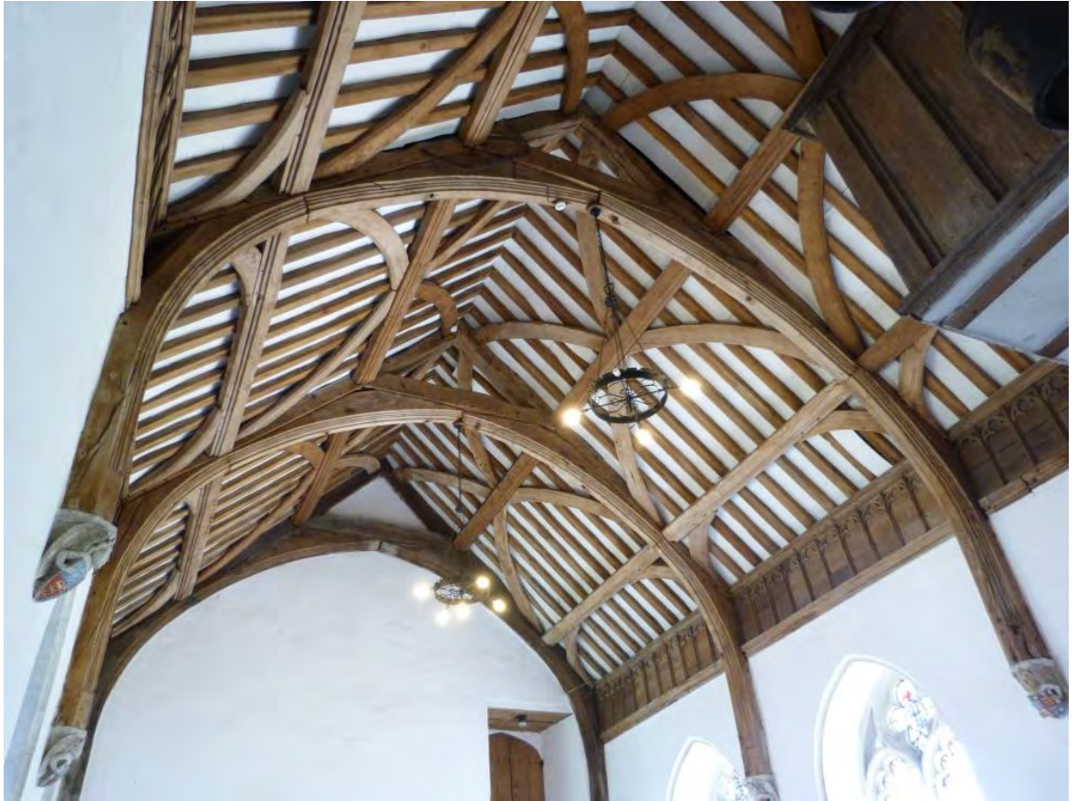
Fig. 3.11: Arch-braced collar roof in the hall of St Cross Hospital, Winchester, 1444 ± 7d.
