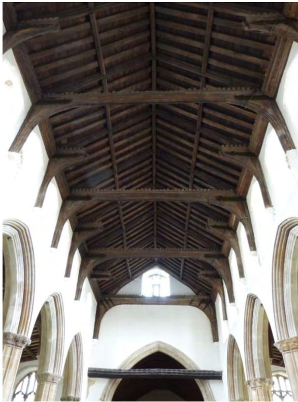
Fig. 8.7: Type 1.2 tie-beam / hammer-beam roofs. Left: Debenham Church, Suffolk, 1403 \pm 6d; right: Bildeston Church, Suffolk, c. 1420.
