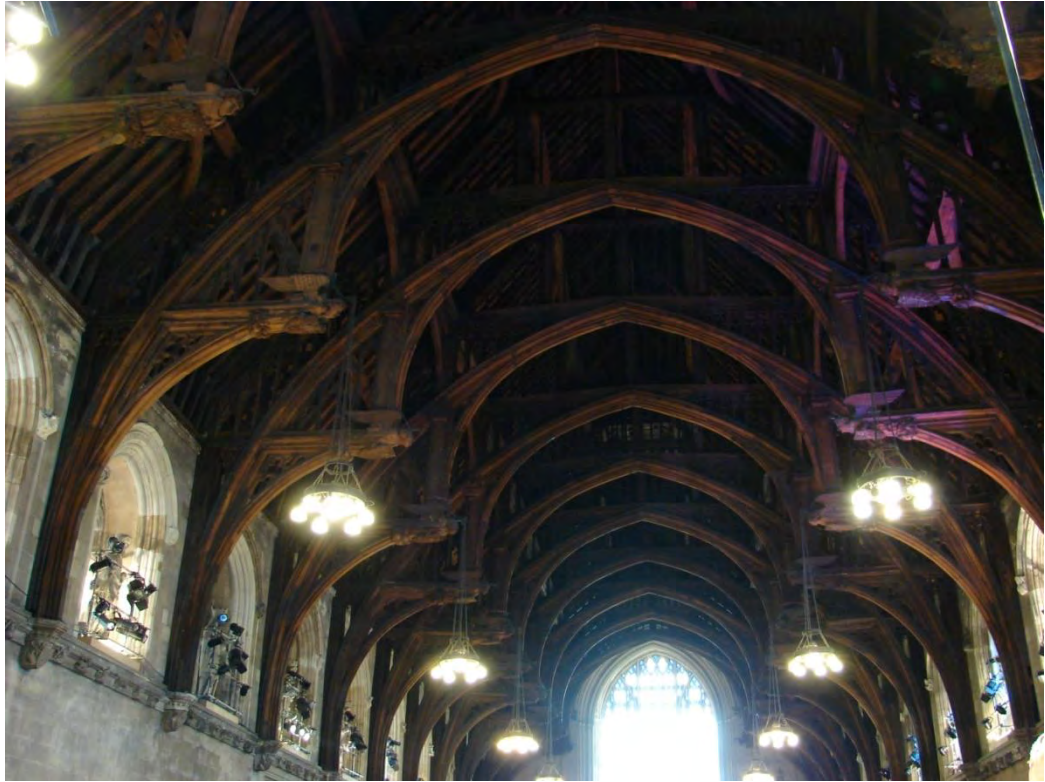
Fig. 5.22: The hammer-beam roof of Westminster Hall, Hugh Herland, begun 1393.
