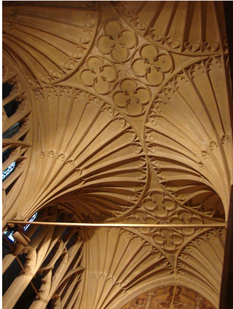
Fig. 1.41: Diminutive early fan vault: Tewkesbury Abbey, The Edward Despenser Chantry, 1375. Note the full extension of the rims of the conoids due to the square-plan bays. Span: 1.66 metres.
