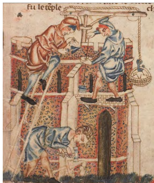
Fig. 4.5: Medieval lifting device, c. 1327-35 (British Library, Add MS. 47682, fol. 27.r)
