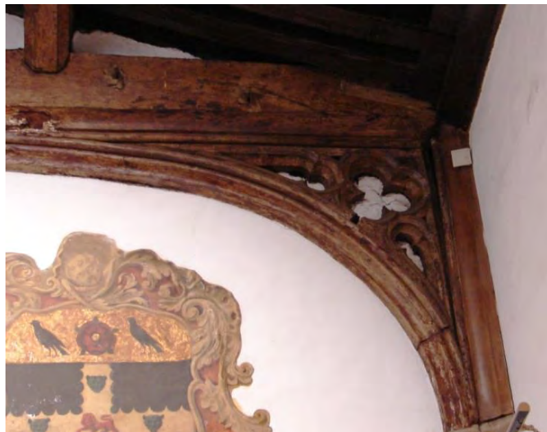
Fig. 6.4: Top: Winchester College, detail of hall wall-post framing. Below: Abbot's Hall, Westminster, c. 1376, detail of same.
