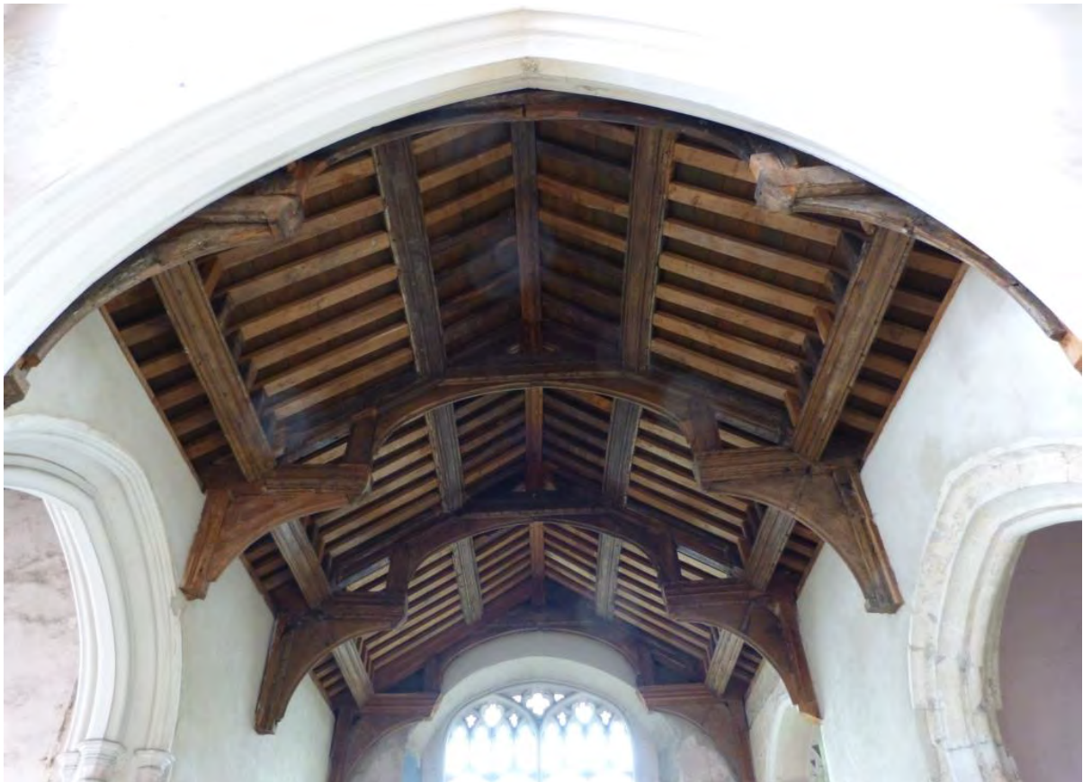
Fig. 3.26: Extended sole piece construction in a hammer-beam roof, St Mary at Quay, Ipswich, chancel, mid fifteenth-century.
