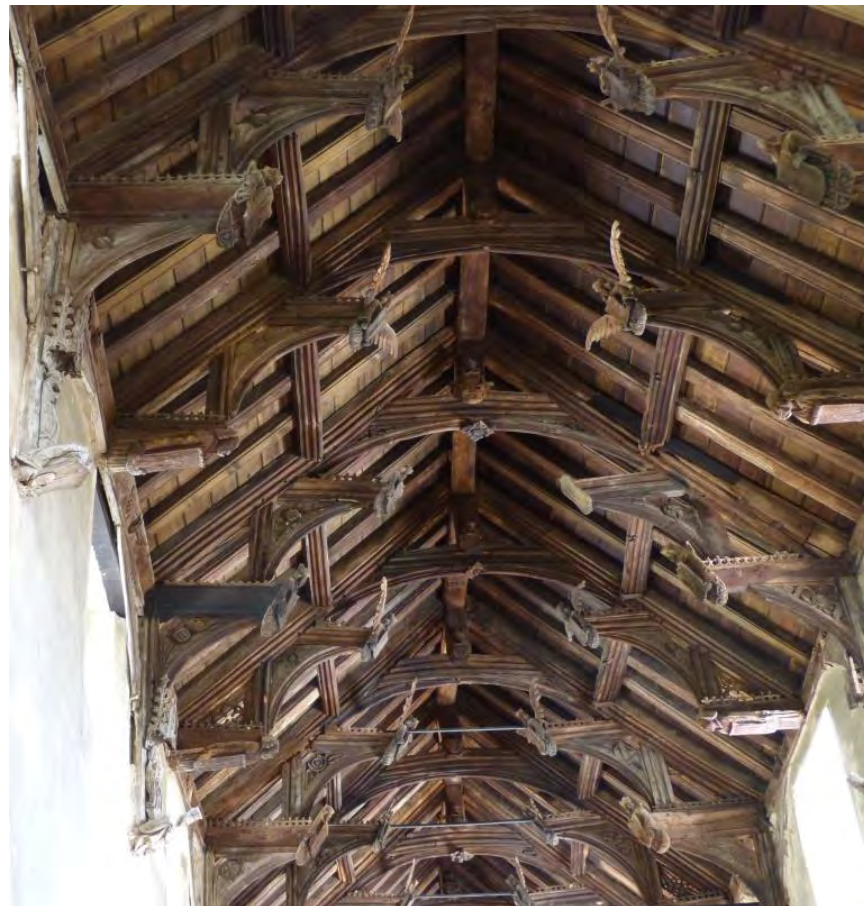
Fig. 2.17: Tilney All Saints Church, fifteenth-century, Norfolk. 'False' double hammer-beam carpentry in the upper tier of hammer beams. Visible are the metal tie-rods inserted to rectify the poor capacity of this structure to counteract lateral thrust.
