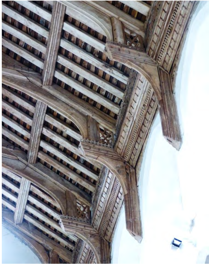
Fig. 6.34: Fressingfield Church, Suffolk, detail of nave roof, fifteenth-century. Note the absence of corbels, but interestingly, the presence of mortices from which suspended corbels may once have been framed.
