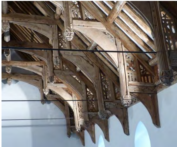
Fig. 1.47: Pendant post hammer-beam roofs. Clockwise from top left: Cotton Church Suffolk, c. 1471 (with alternate arch-braced frames); Wetherden, Suffolk; Grundisburgh; Suffolk (pendants are in the upper tier of hammer posts), both probably late fifteenth-century. Gestingthorpe Church, Essex, 1489. All double hammer-beams.
