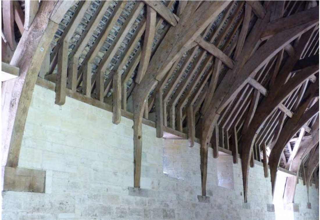
Fig. 3.21: Extended Ashlars in situ , Bradford on Avon Tithe Barn, Wiltshire, 1334-79d.
