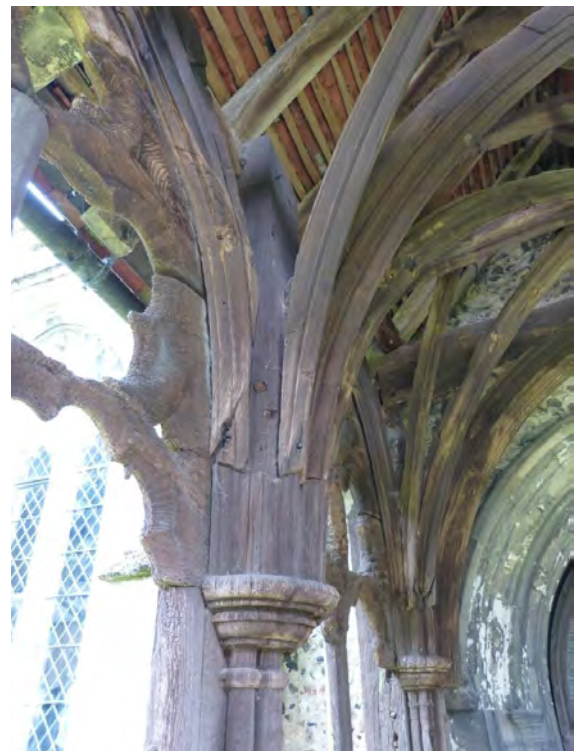
Fig. 6.6: Boxford Church, Suffolk, timber north porch, fourteenth-century; right: detail of wall post to rib framing.
