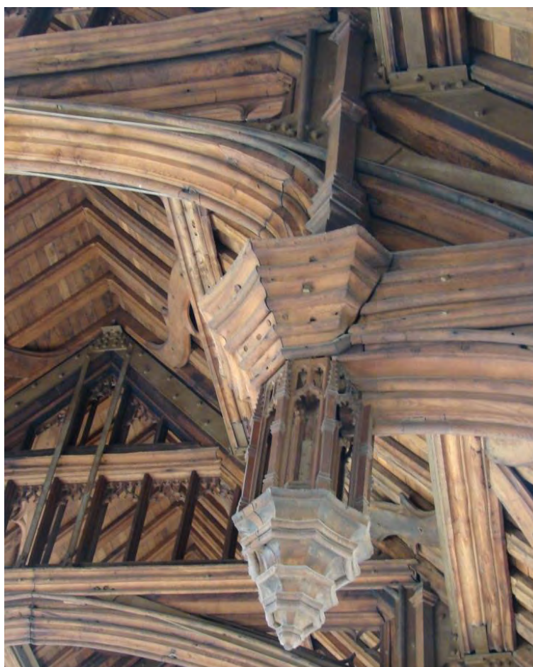
Fig. 8.40: Eltham Palace, detail of pendant hammer post.
