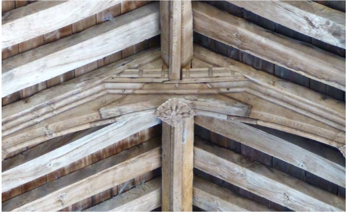
Fig. 8.47: Great Cressingham, nave roof, detail of apex framing.
