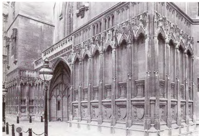
Fig. 5.19: Westminster Hall, north facade, statuary arcading. Compare Fig. 5.22 below. (Wilson/RCHME)
