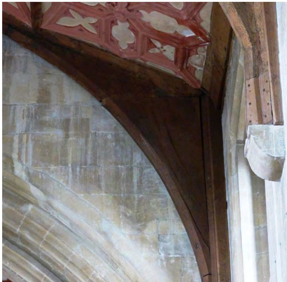
Fig. 3.8: Edington Church, Wiltshire. Top: nave, looking east; below: detail of jointed arch brace. The main structure of the church dates to the mid fourteenth century, but the date of the roof is uncertain.
