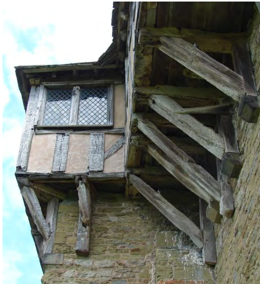
Fig. 3.28: Medieval bracketed structure: jettying on north tower, Stokesay Castle, c. 1290. Interestingly, a number of these brackets have no corbels.
