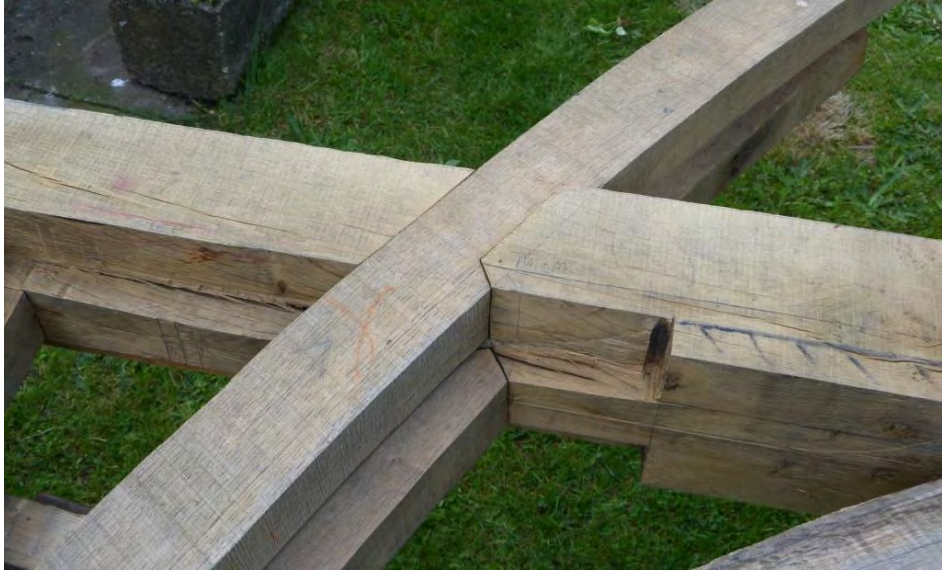
Fig. 6.26: Reconstruction of Westminster framing, note narrowing of the laminate as it passes through the hammer beam.
