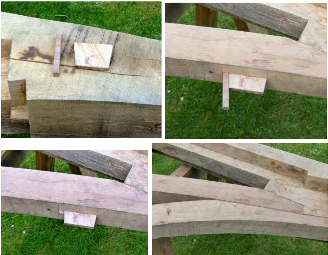
Fig. 6.33: Reconstruction of Westminster framing, assembly procedure for dovetailed key at the conjunction of core / curved strut. Top left: key and packing piece prepared. Top right: inserted into mortice in core (the packing piece remains to be trimmed). Lower left: packing piece trimmed; the key cannot now be withdrawn (the peg hole cannot be bored until the joint is assembled). Lower right: joint assembled and pegged through curved strut.
