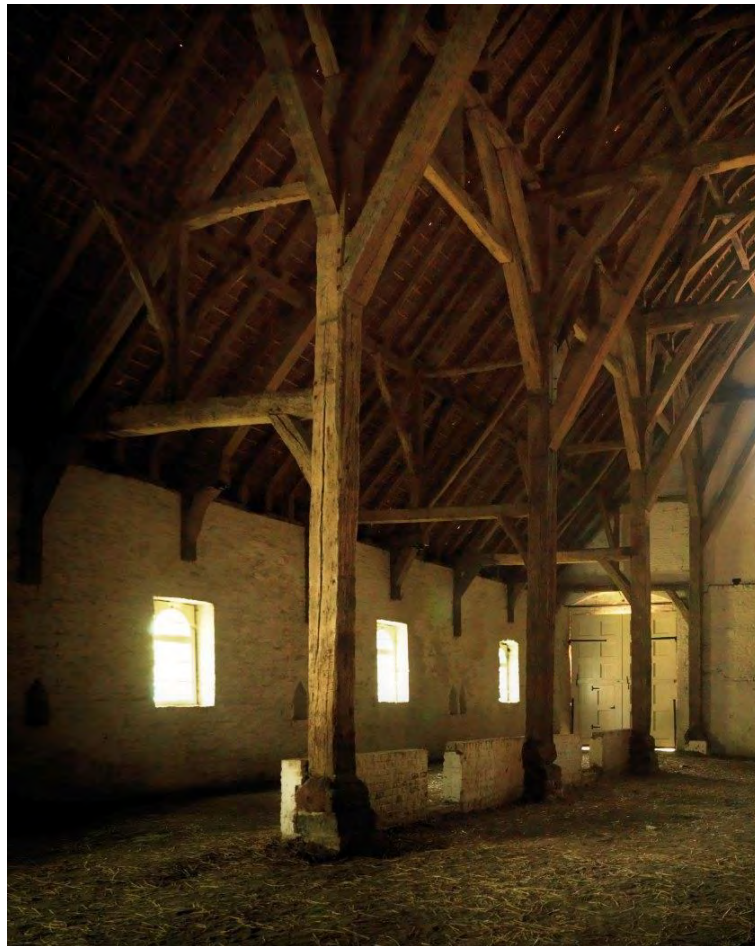
Fig. 4.15: Aisle tie and hammer-beam framing, barn, Ter Doest Abbey, Lissewege, Belgium, 1365-85d. ( http://visitbruges.be )
