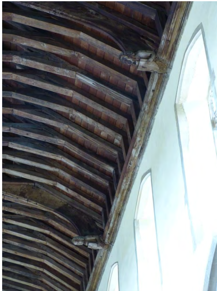
Fig. 3.24: Example of extended sole piece construction, Wingfield Church, Suffolk, nave, c. 1415. The internal 'wall plate' is a moulded cornice.
