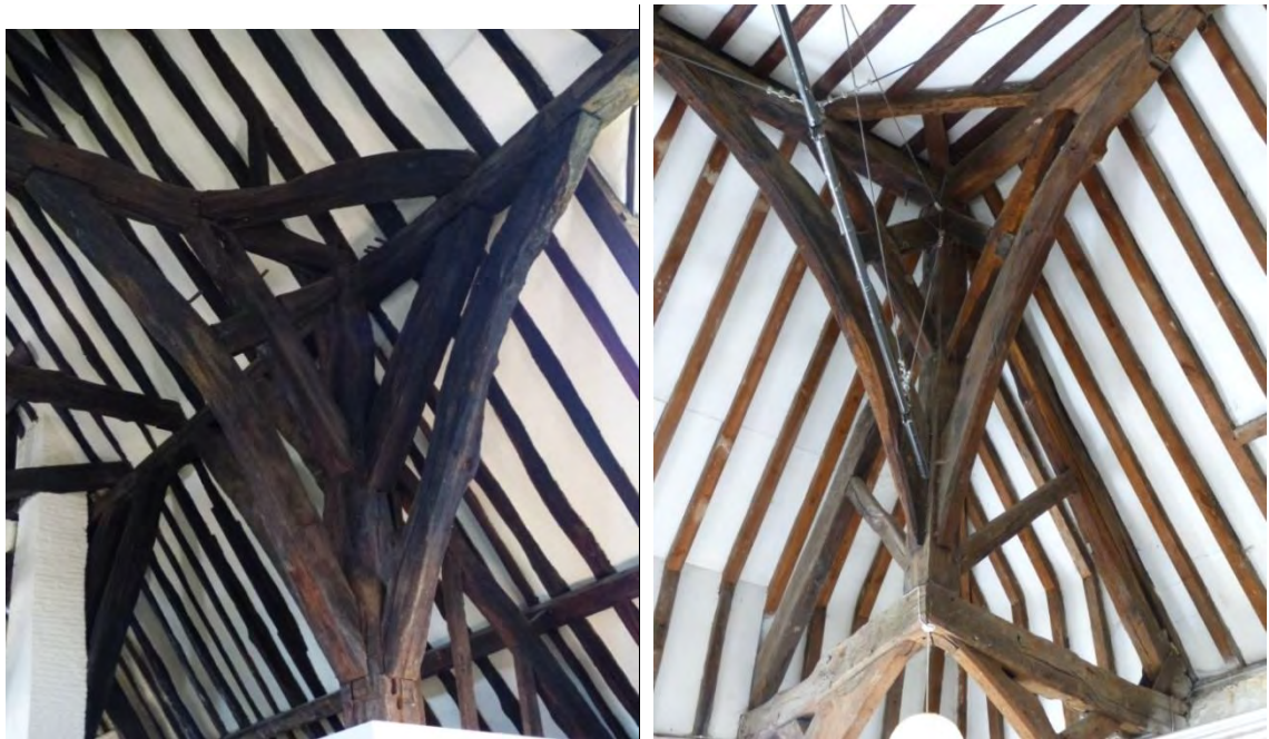
Fig. 4.31: Late thirteenth-century Chichester Carpentry. Left: St Mary's Hospital, arcade post framing; Right: Bishop's Kitchen, hammer-beam arrangement
