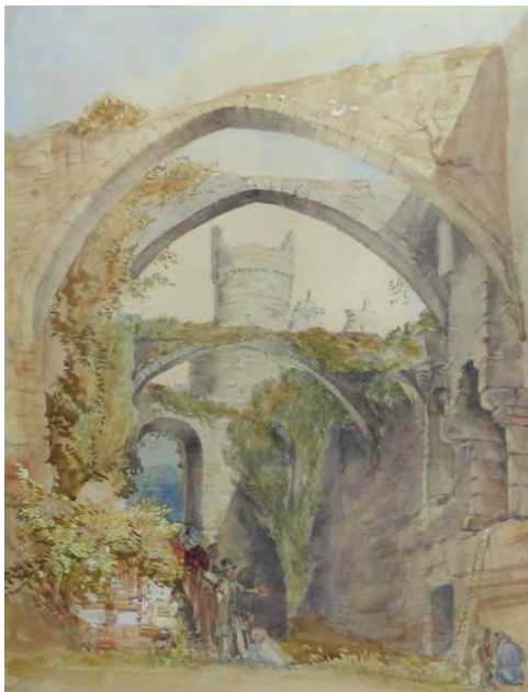
Fig. 7.4: Conway Castle, North Wales, great hall c. 1346, remains of roof. Left: mid-19 th century watercolour by J. H. Pollen. By the 20 th century only one arch remained, but note the springing points of the lost arches.
