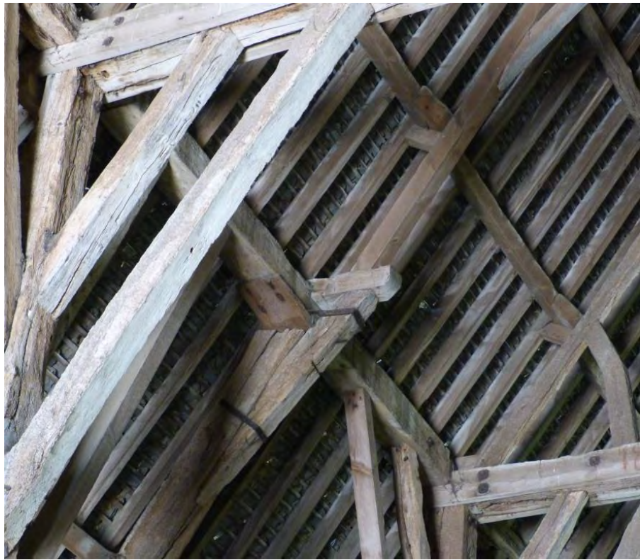
Fig 4.17: Great Coxwell Barn, 'germinal ... hammer-beam', detail of framing in intermediate frame.
