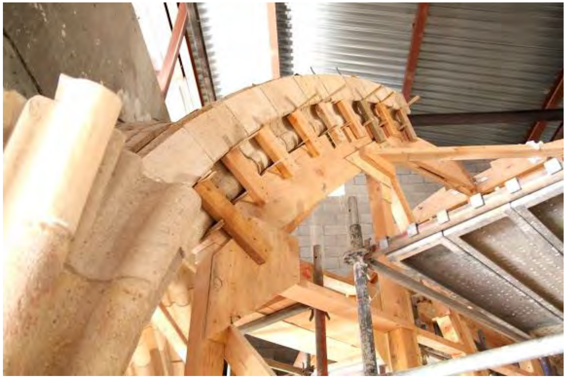
Fig. 1.21: Abbey of New Clairvaux. Note the wedges for fine adjustment of the voussoirs.
