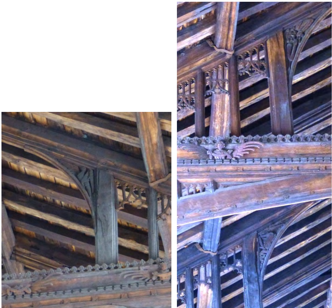
Fig. 8.3: King's Lynn, St Nicholas, details of roof showing carved spandrels of queen-post braces.
