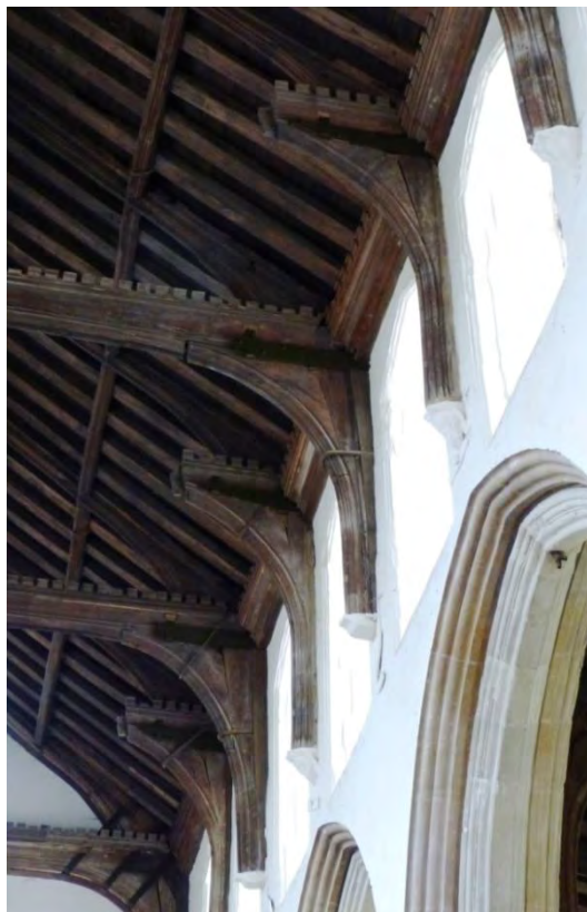
Fig. 8.8: Left: Debenham Church, note extant tenons on ends of hammer beams; right: Bildeston Church, replaced hammer-beam angels.
