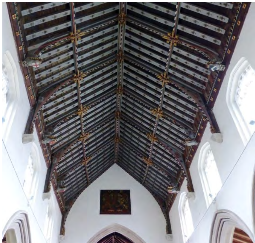
Fig. 8.22: The perfect carpentered Gothic arch? Northwold Church, Norfolk, nave, fifteenth-century. The hammer beams are non-structural; the roof is of arch-braced principal construction.
