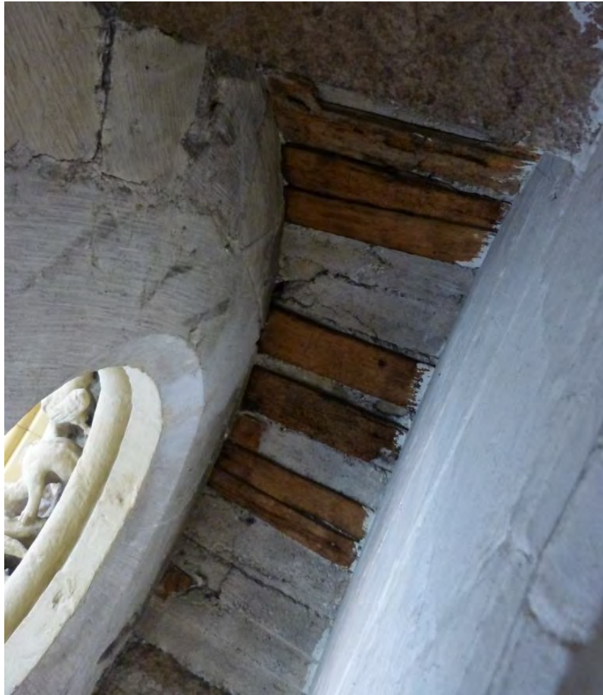
Fig. 1.17: Boards inserted to support an area of vault webbing, Chichester Cathedral, choir gallery.
