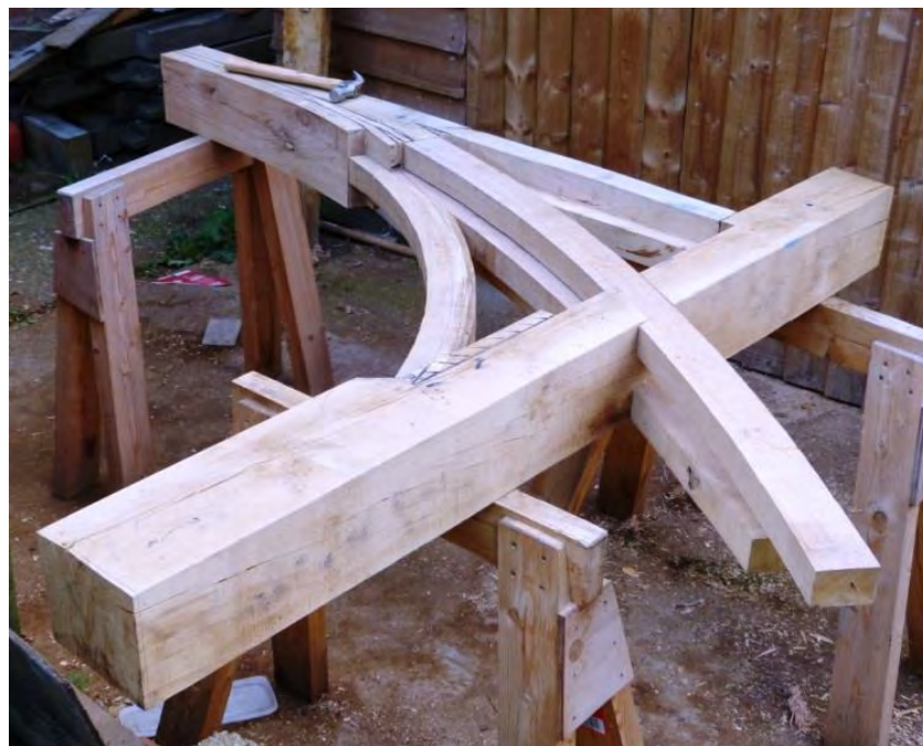
Fig. 6.1: Reconstruction of Westminster Hall lower framing at scale of 1:4 in green oak (Robert Beech & Chris Dalton)
