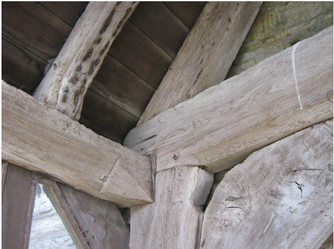
Fig. 2.5b: Normal assembly, porch at Hartpury Church, Worcs., probably fourteenth-century.
