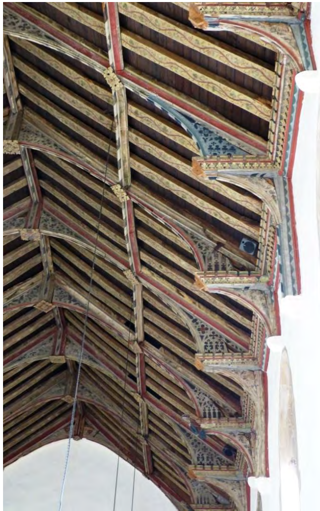
Fig. 8.42: Bardwell Church, Suffolk, detail of nave roof, c. 1421. Note tenons to which hammer-beam angels were once fixed; note also king pendant construction at apex.
