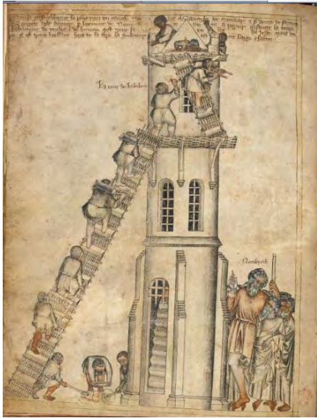
Fig. 4.1: Fourteenth-century scaffolding, and detail. (British Library, Egerton MS. 1894, fol. 5v.)
