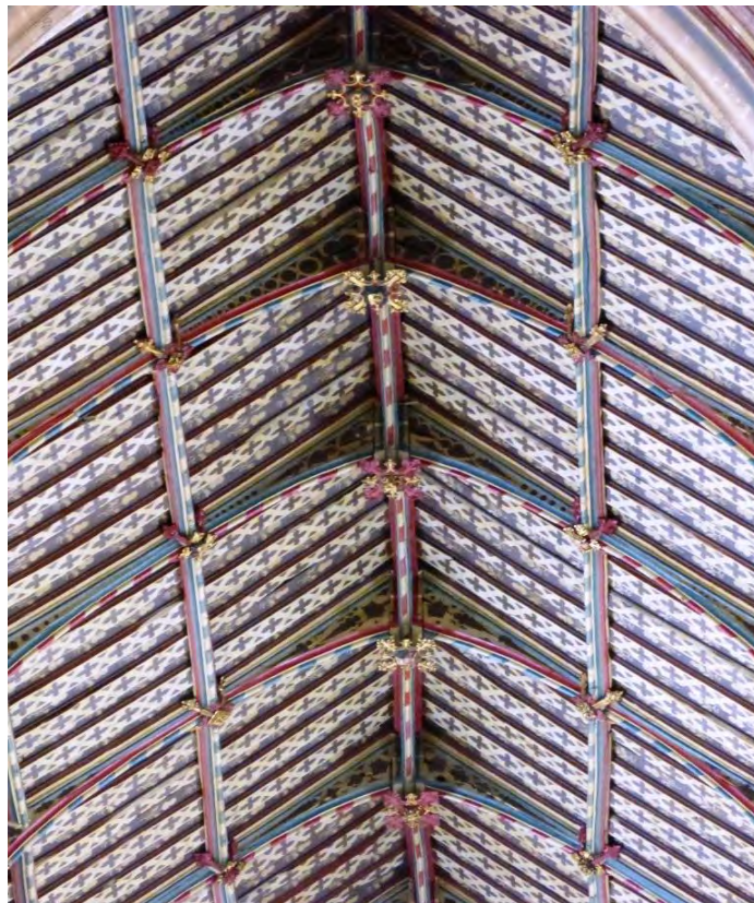
Fig. 8.15: King pendant construction, apex framing, Ely Cathedral, north transept.
