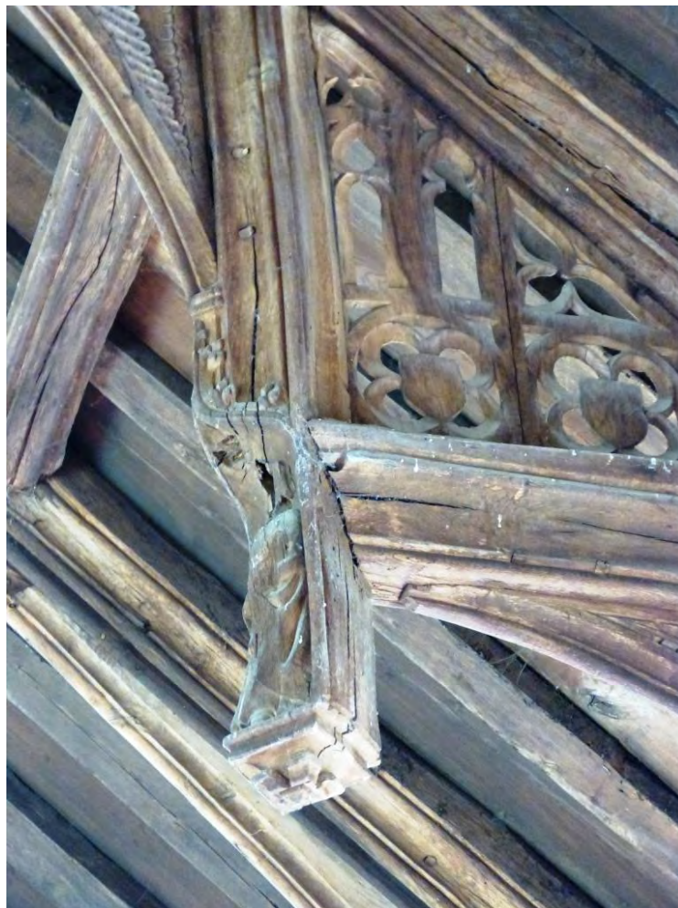
Fig. 8.38: Tostock Church, nave roof, detail of lower pendant post.
