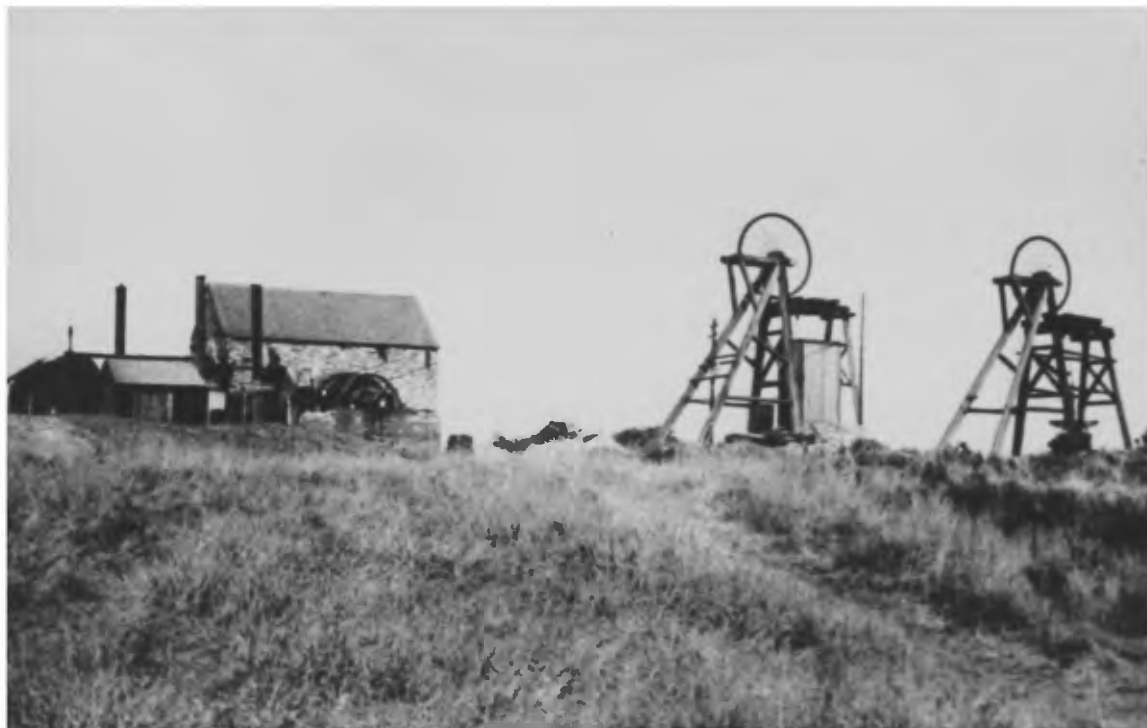
Colliery at Upper Gornal, Sedgley, in the South Staffordshire Coalfield. Pithead gear at one of the small collieries still working in the western part of the Conurbation. Lifts and cages have improved upon the simple pithead gear of the nineteenth century, and beam engines have been replaced by more efficient steam engines, but in many cases a century has produced few essential changes in mining methods and pithead equipment.
