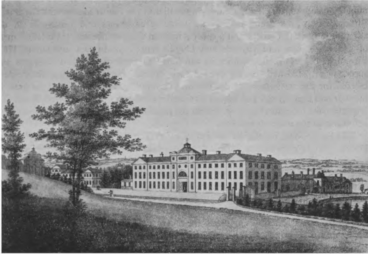
The Soho Manufactory as it appeared at the end of the eighteenth century.
