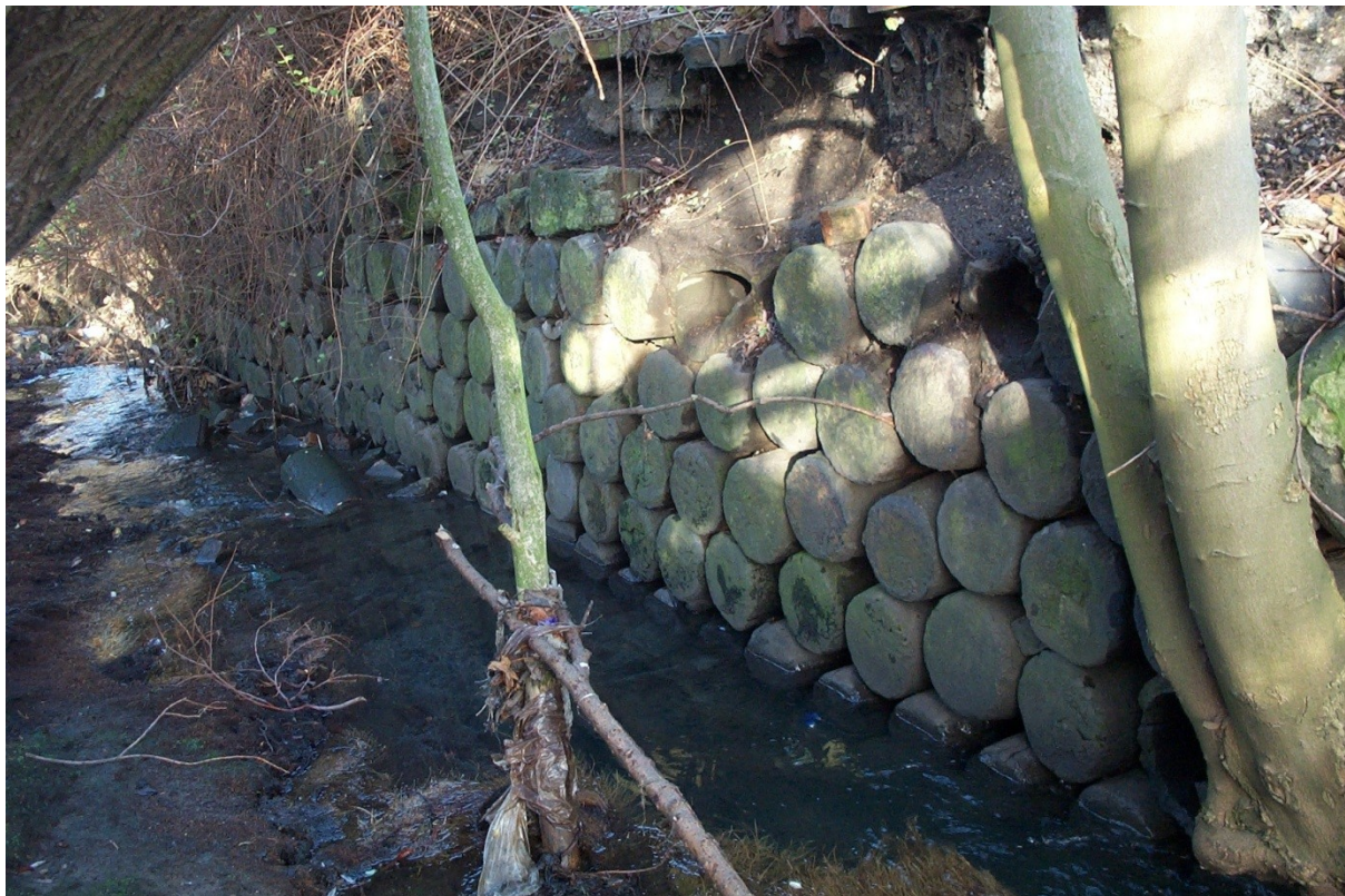
Figure 50 Spent phosphorus retorts from Albright and Wilson used as a wall in Langley brook 94
