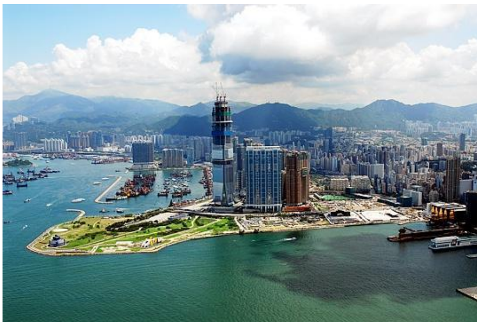
Pic. 4.1 West Kowloon Cultural District (WKCD), HongKong
