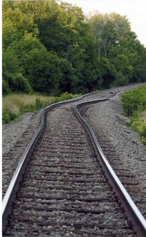
Figure 2.3: Example of a buckle on curved track (TSB, 2002)
