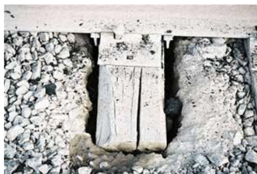
Figure 2.4: Example of subgrade contamination of ballast and the resulting reduced support offered by the ballast to the sleeper (TSB, 2003)
