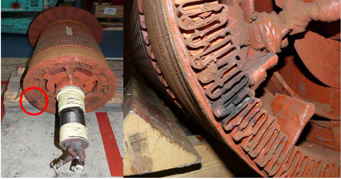
Figure 7.18: Generator rotor winding failure
