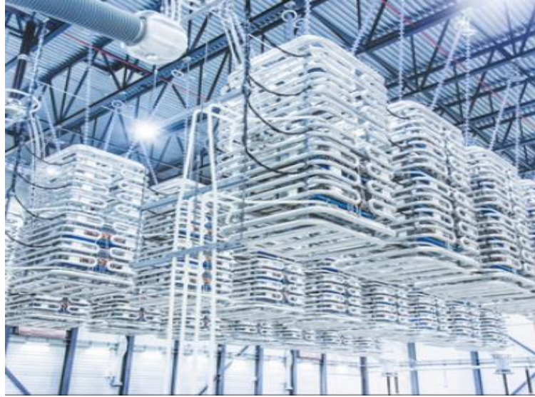
Fig. 1.4 A photo of sub-modules forming a multilevel converter [25].
