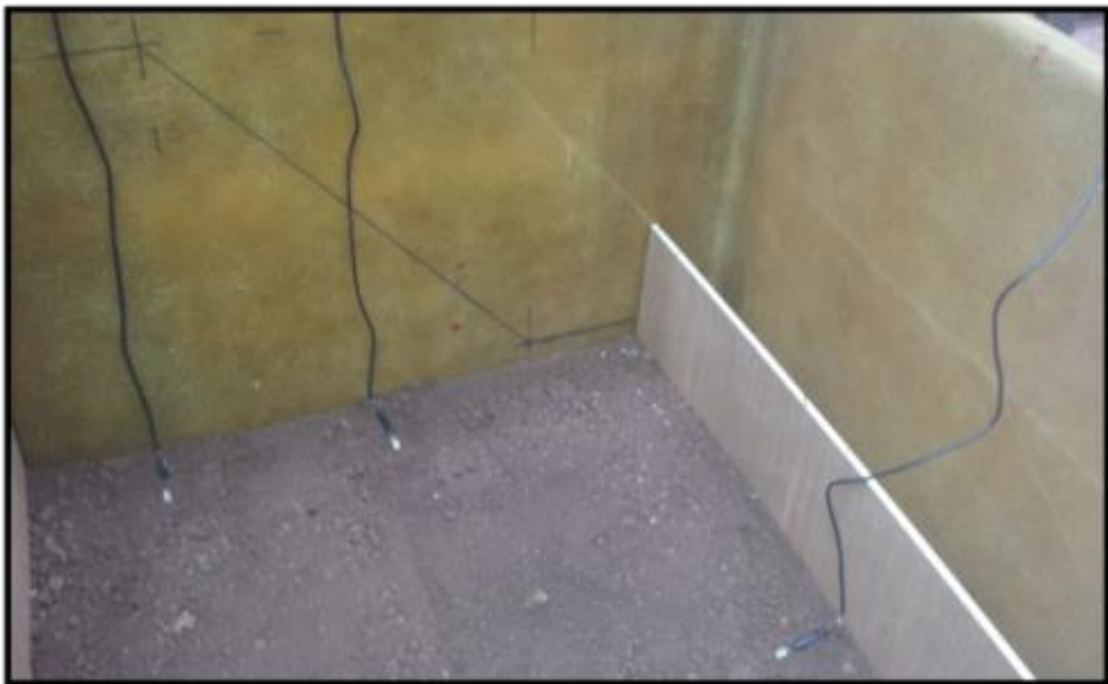
Figure 5-32: Burying MPS-6 sensors during slope construction
