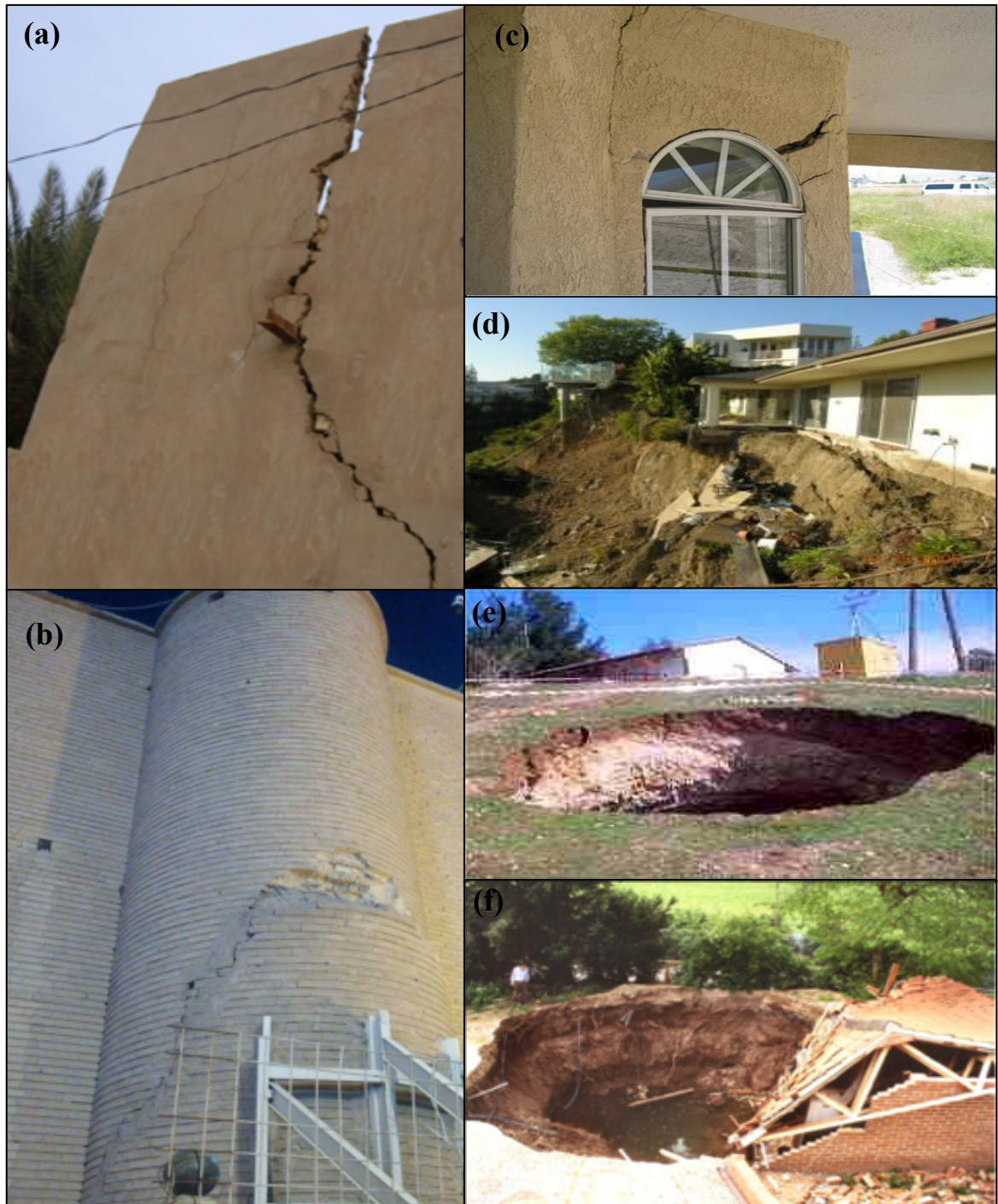
Figure 1-1: (a) and (b) Cracks in the walls of a house and historical building (rebuilt three years ago), respectively, due to differential settlement from Al-Najaf city, Iraq (by the author, 2017), (c) and (d) Differential settlement and collapse in a house in Iraq (Awn, 2010), (e) Sinkhole, 500 m downstream from Mosul Dam in Iraq (Salih, 2013), (f) Sinkhole at Ure Bank Terrace, Ripon, UK; the hole formed in April 1997, 10 m across and 5.5 m deep (Cooper, 2007).
