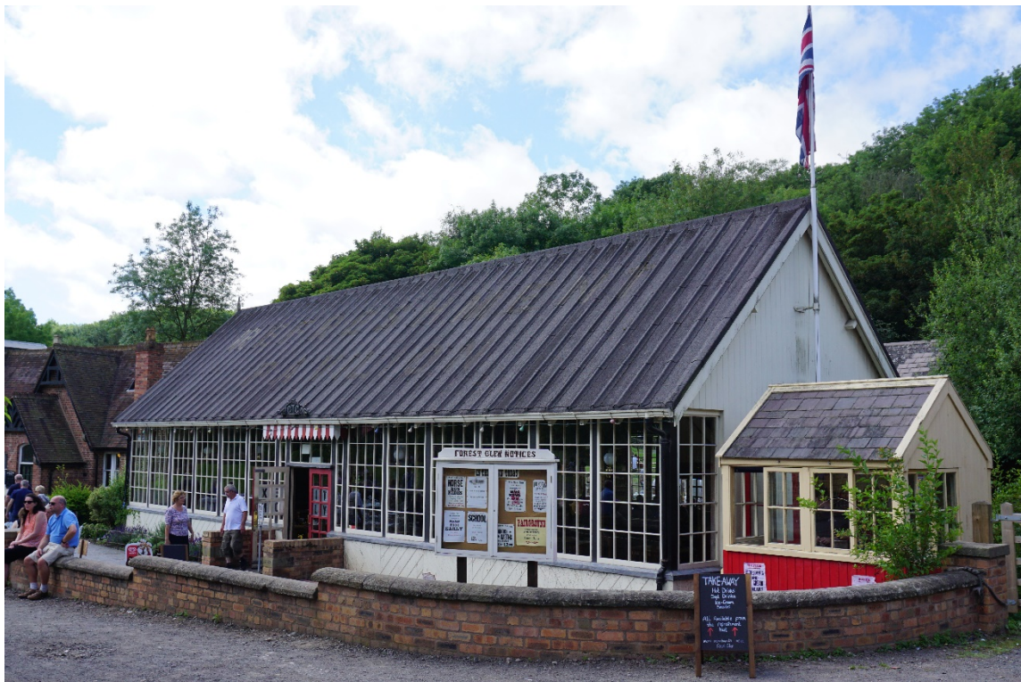
Figure 9. Forest Glen in Blists Hill, relocated building. ©Author
