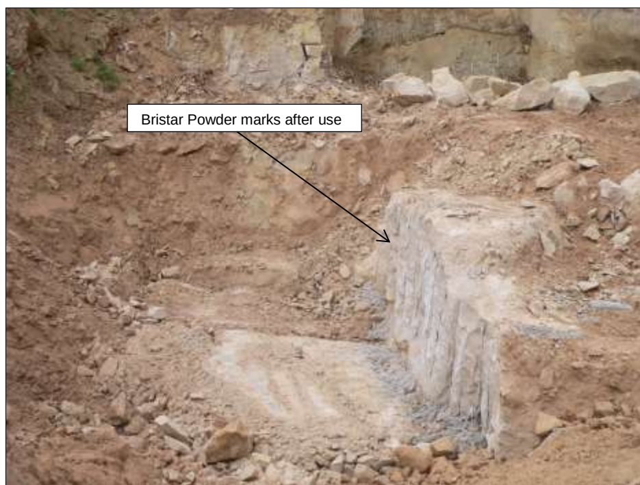
Figure 6: Showing stone site after stone block removed. Taken by author 10/08/2011.
