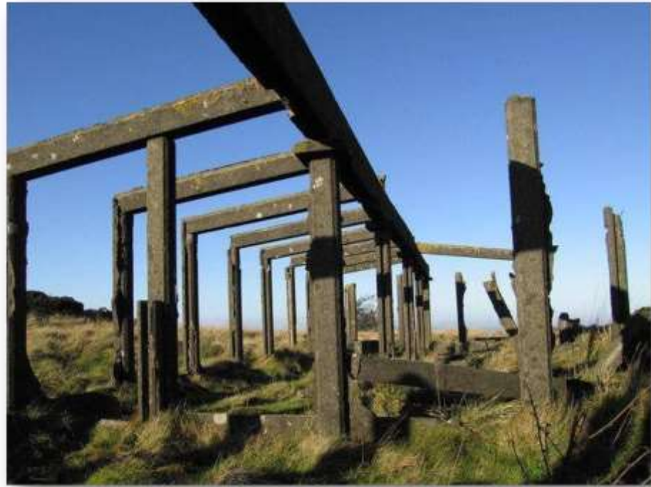
Figure 5.19: Frame of old quarry building on Abdon Burf, on Abdon Clee Hill, Shropshire (Source: www.geolocation.ws , accessed 12/04/2013).
