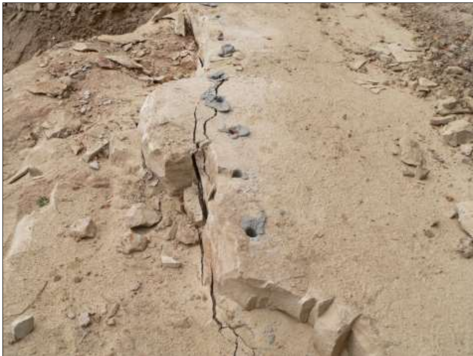
Figure 4: Holes where Bristar Powder was drilled and placed. Taken by author 10/08/2011.
