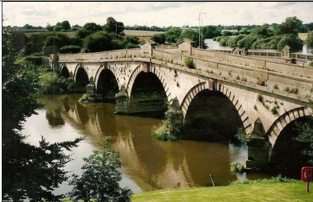
Figure 3. 3: Atcham Bridge. (Source: www.bing.com/images/search?q=Atcham+Bridge+shrewsbury accessed 23/08/2016).
