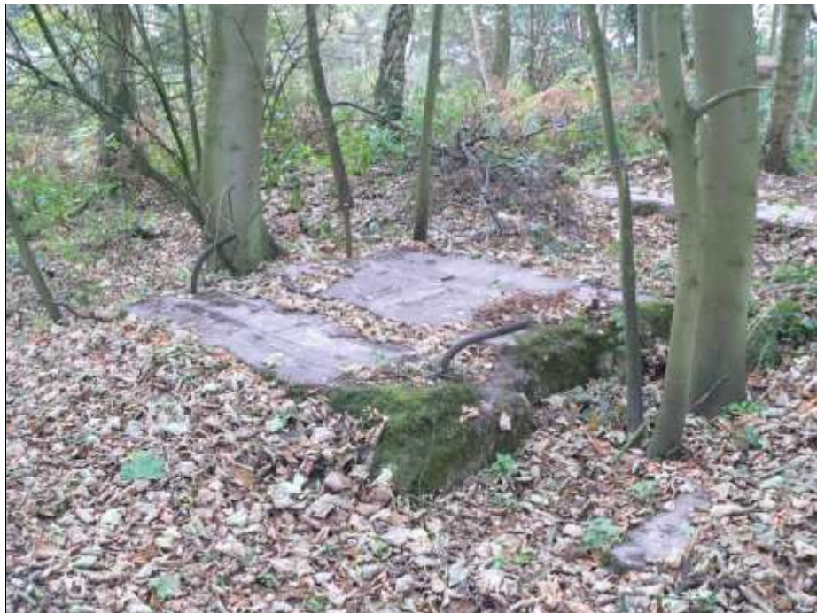
Figure 2: Grinshill Stone Quarries, former crane foundations. Taken by author: 10/08/2011
