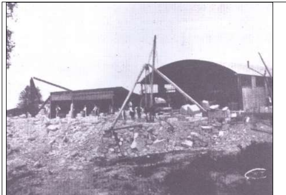
Figure 3.7: The above picture above shows men working in the sheds possibly dressing stone; other men are working with a wooden crane which lifts stone blocks. Source: The Grinshill Quarries from their heyday in Victorian times until 1923 (Thomson, 2004).
