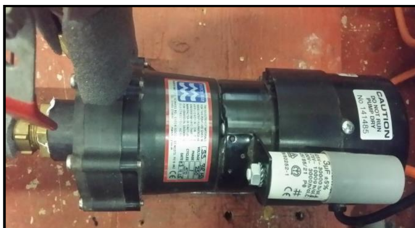
Fig. 7-6 Chilled water pump.
