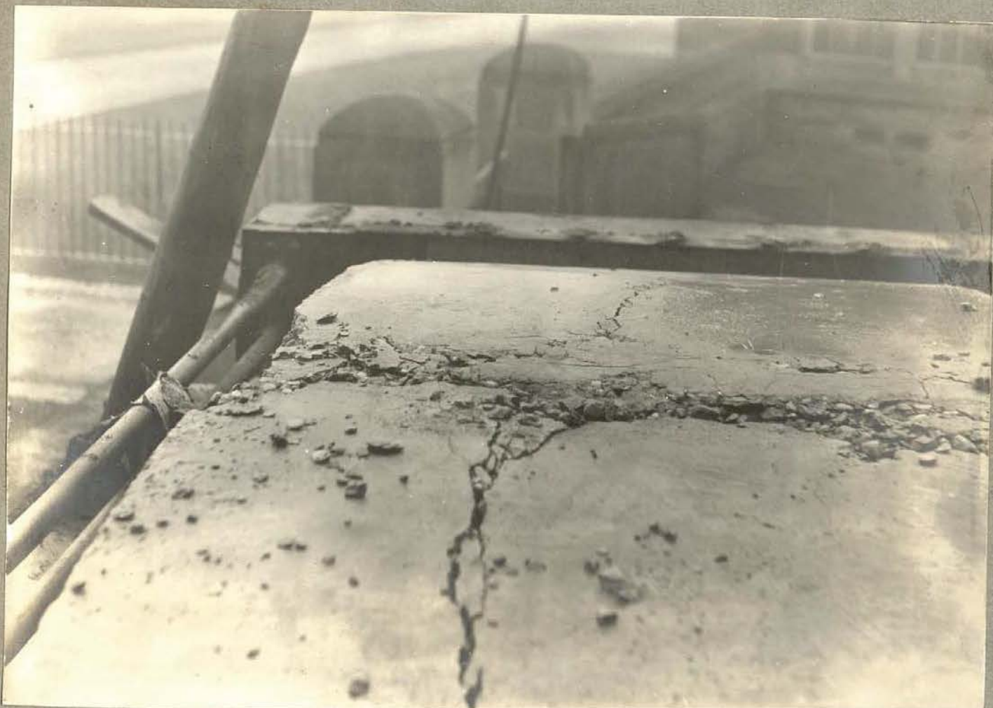
FRACTURE OF ARCH No.1.
