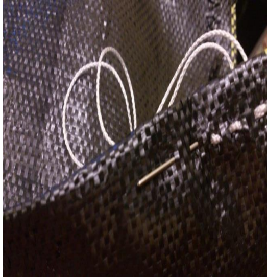
Figure 4.13: Stitching the geotextile to form a cylinder encasement
