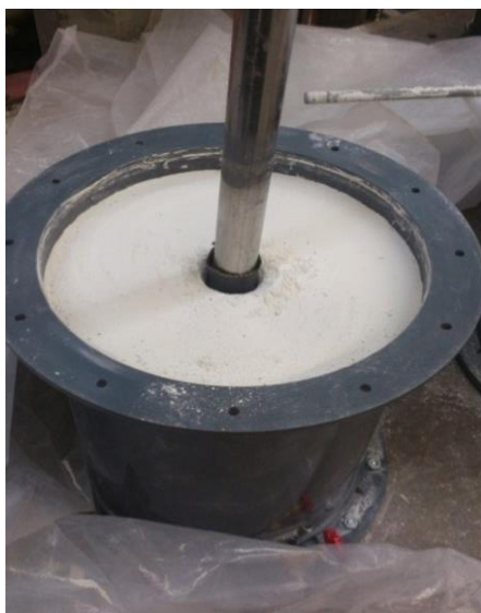
Figure 4.12: Wrapping the geotextile around the steel tube
