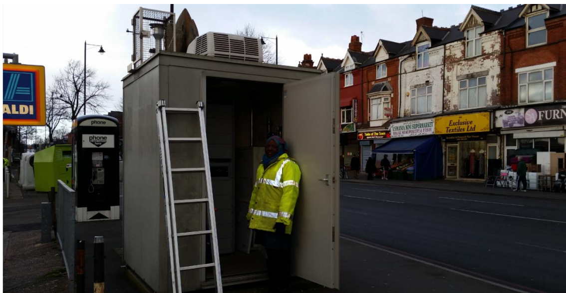
Figure 14 Samplers kept in cabin owned by Birmingham city council with inlets placed on the roof of the cabin.
