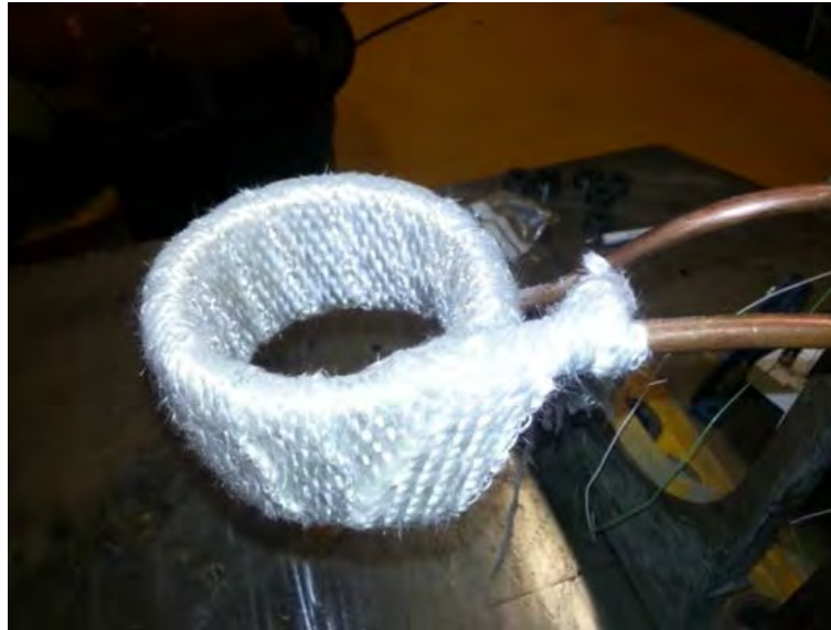
Figure 3-6 - Induction coil with glass fibre insulation in place.
