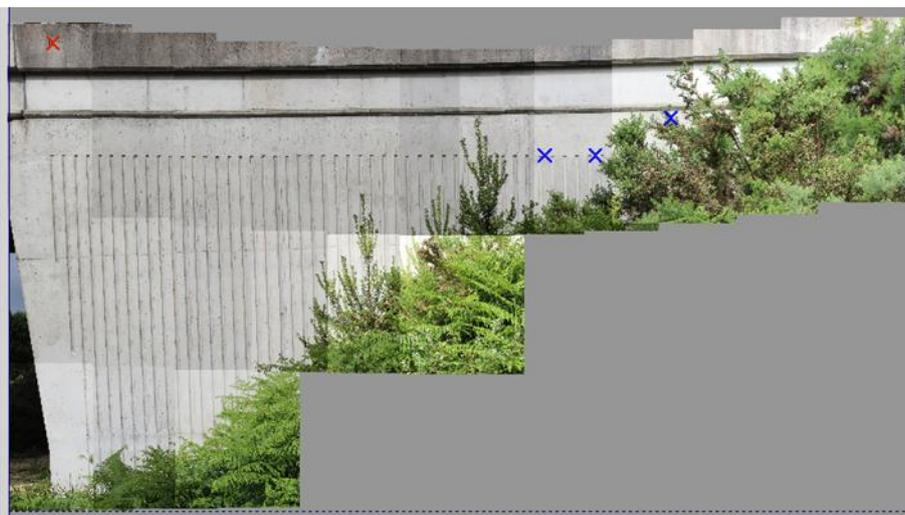
**Figure 131: Defect map overlaid on tessellated imageset from IP5.**
