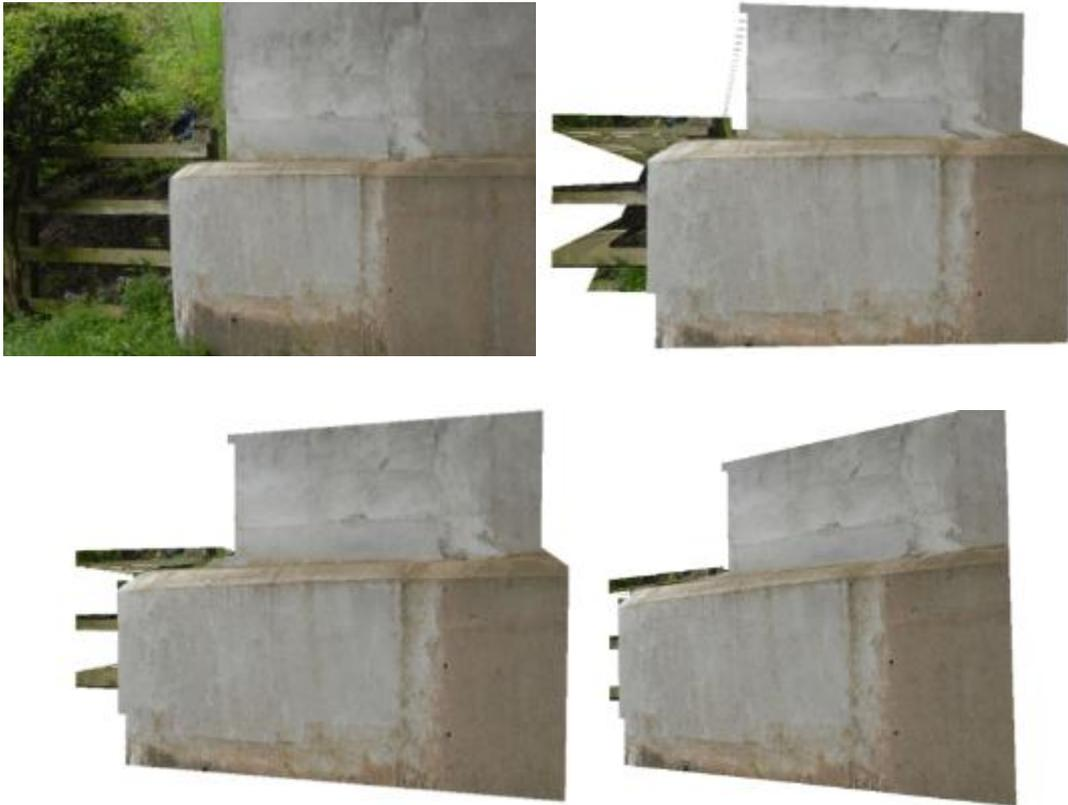
**Figure 119: Original 2-D image data (top left) and three views of 3-D representations created from this image data and artificial LiDAR shape measurement data.**
