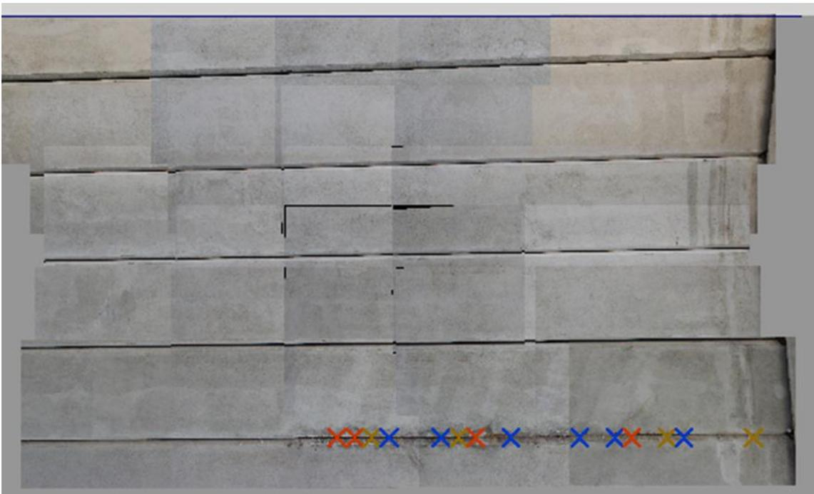
**Figure 136: Defect map overlaid on tessellated imageset from IP11.**
