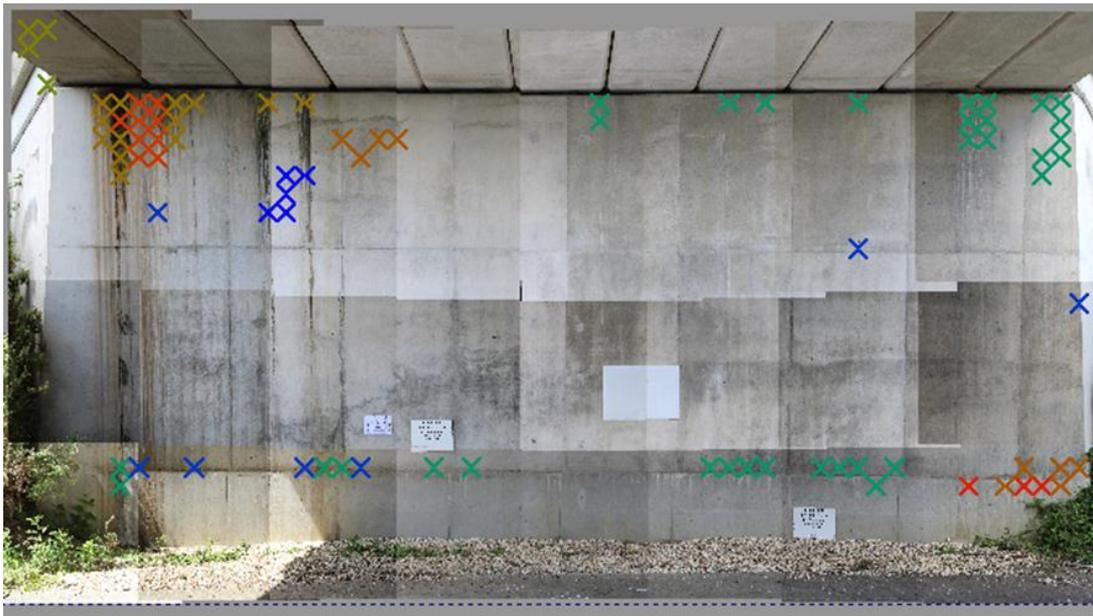
**Figure 127: Defect map overlaid on tessellated imageset from IP1.**
