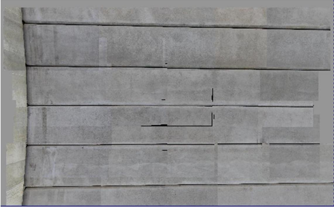
**Figure 137: Defect map overlaid on tessellated imageset from IP12.**
