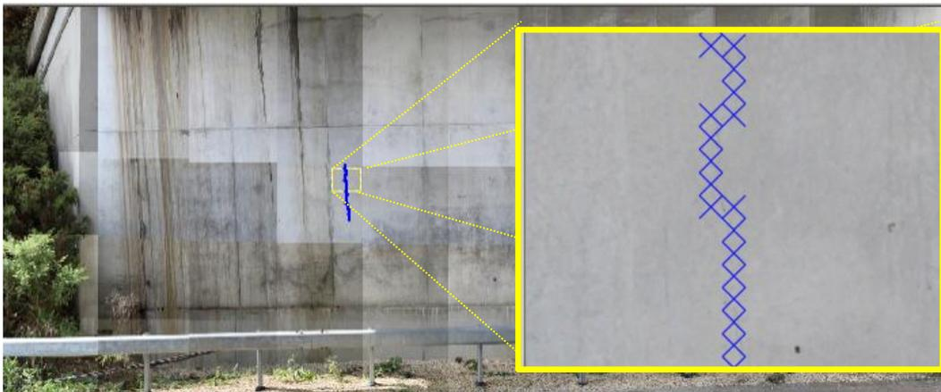
**Figure 94: Tessellated view, with overlaid zoomed in image, showing marked defect location.**
