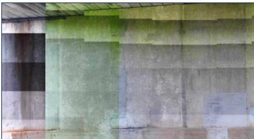
**Figure 91: Example of tessellated images showing large colour and intensity differences due to changing illumination conditions.**
