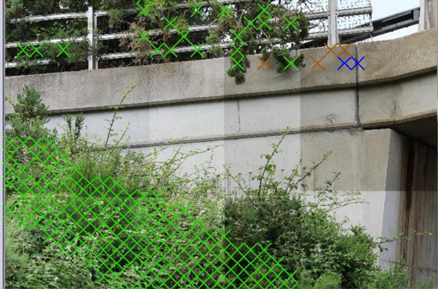
**Figure 129: Defect map overlaid on tessellated imageset from IP3.**
