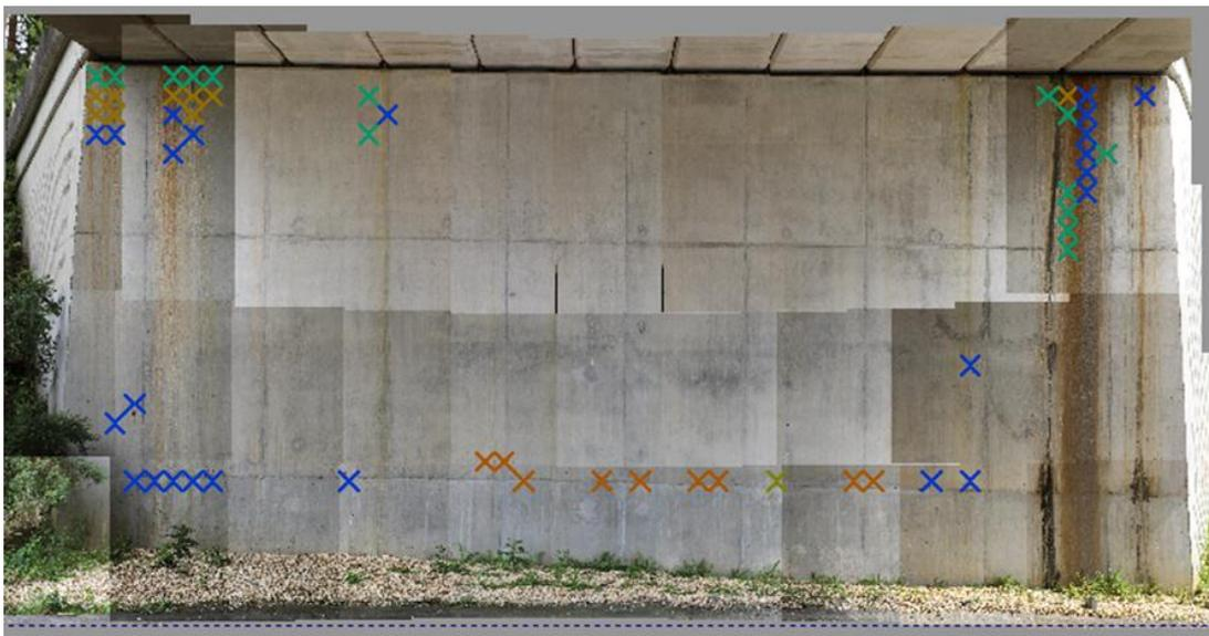
**Figure 128: Defect map overlaid on tessellated imageset from IP2.**
