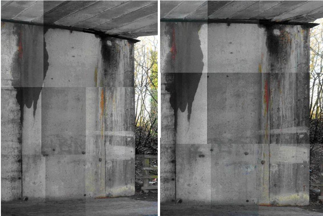
**Figure 85: Example of effect of reprojection - Mosaic of nine un-reprojected images (left) and the same nine images following reprojection (right).**
