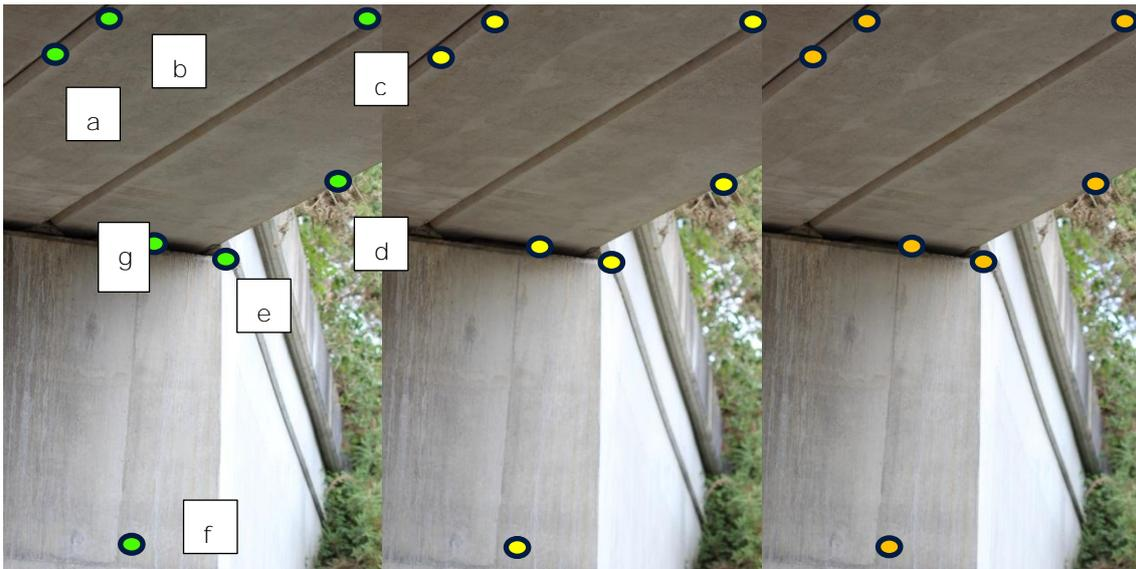
**Figure 114: Three images taken in successive sweeps of bridge surface showing repeatability of positioning.**
