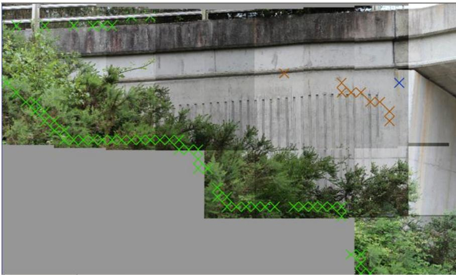
**Figure 134: Defect map overlaid on tessellated imageset from IP8.**
