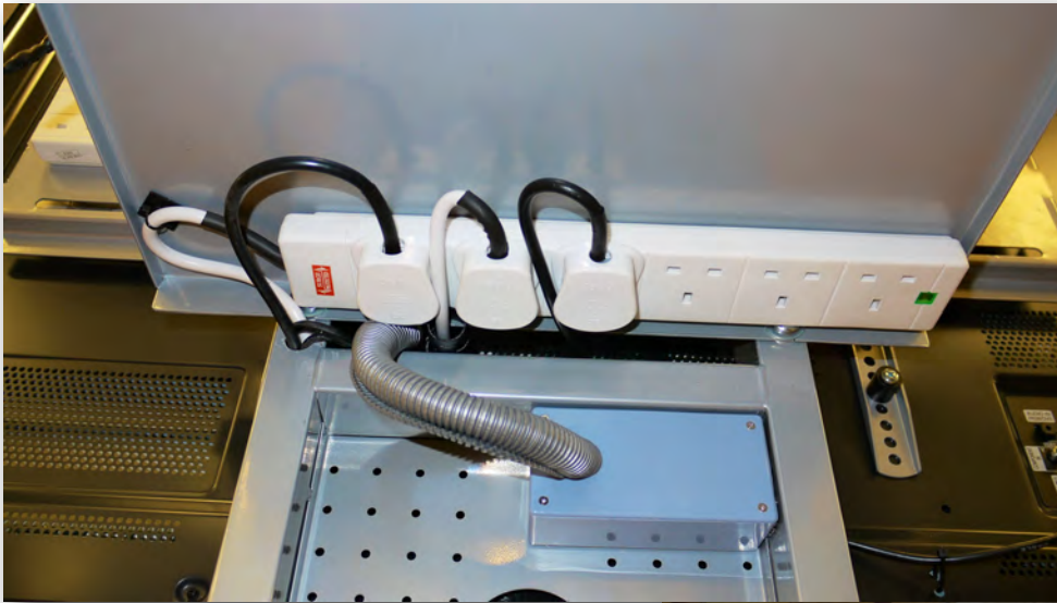
Figure 5.8 Mains block mounted to the underside of the AV shelf.
