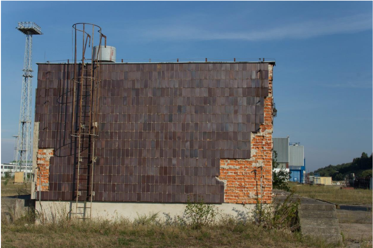
Figure 4.11 (marked ‘D’ in figure 4.1) A gas power plant adjacent to the ruins of Żarnowiec NPP. The facility was constructed in the 1990s but the investment fell through due to a lack of transport infrastructure and the termination of all long term contracts within the Special Economic Zone (PSSE) following EU accession (see Chapter 5).
