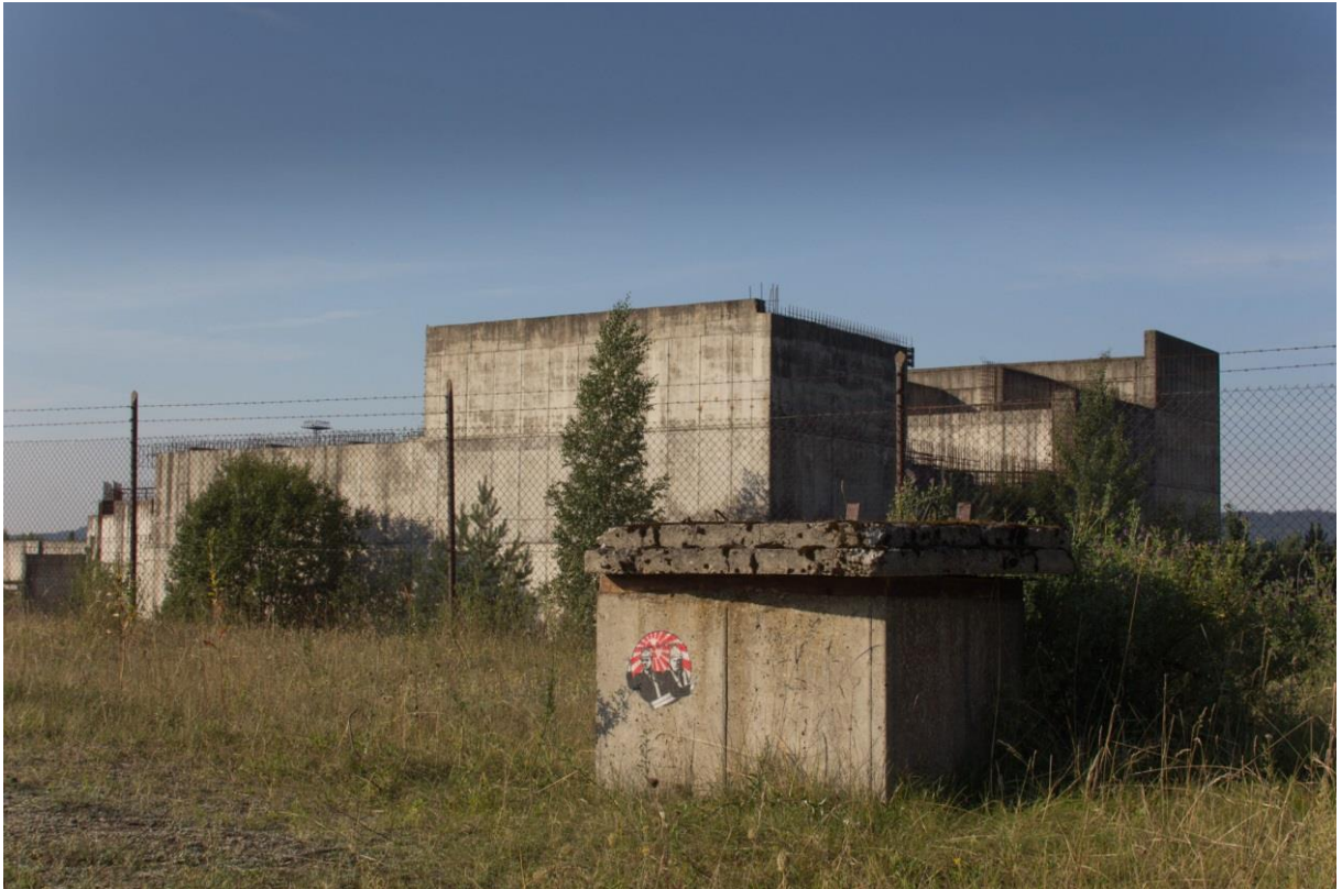
Figure 4.8 (marked 'C' in figure 4.1) A different angle of the abandoned reactor buildings from the 1980s construction of Żarnowiec NPP.
