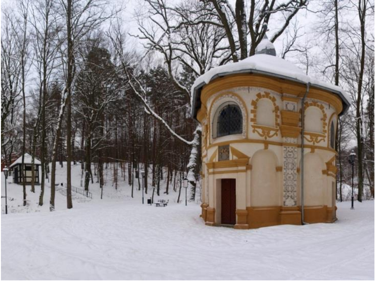
Figure 1.4 Chapels at Kalwaria Wejherowska, on the outskirts of the Kashubian town of Wejherowo. The chapels are on a pilgrimage route which winds through the towns and villages of northern Pomerania during the spring and summer months. (Photograph by author, February 2011)
