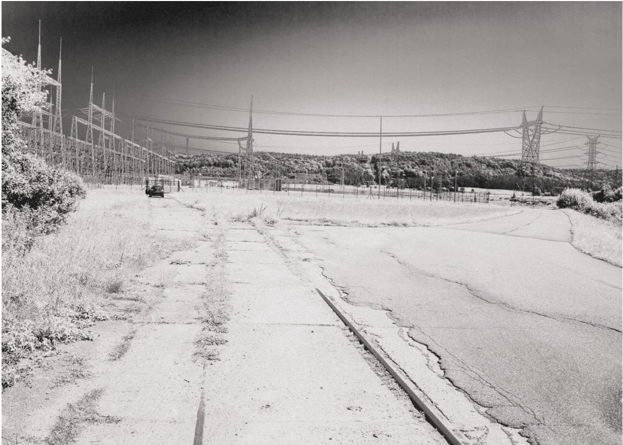
Figure 5.1 The railway station at Żarnowiec is long gone, but the substation and transmission network still hums with activity. (Photograph by author, July 2012)
