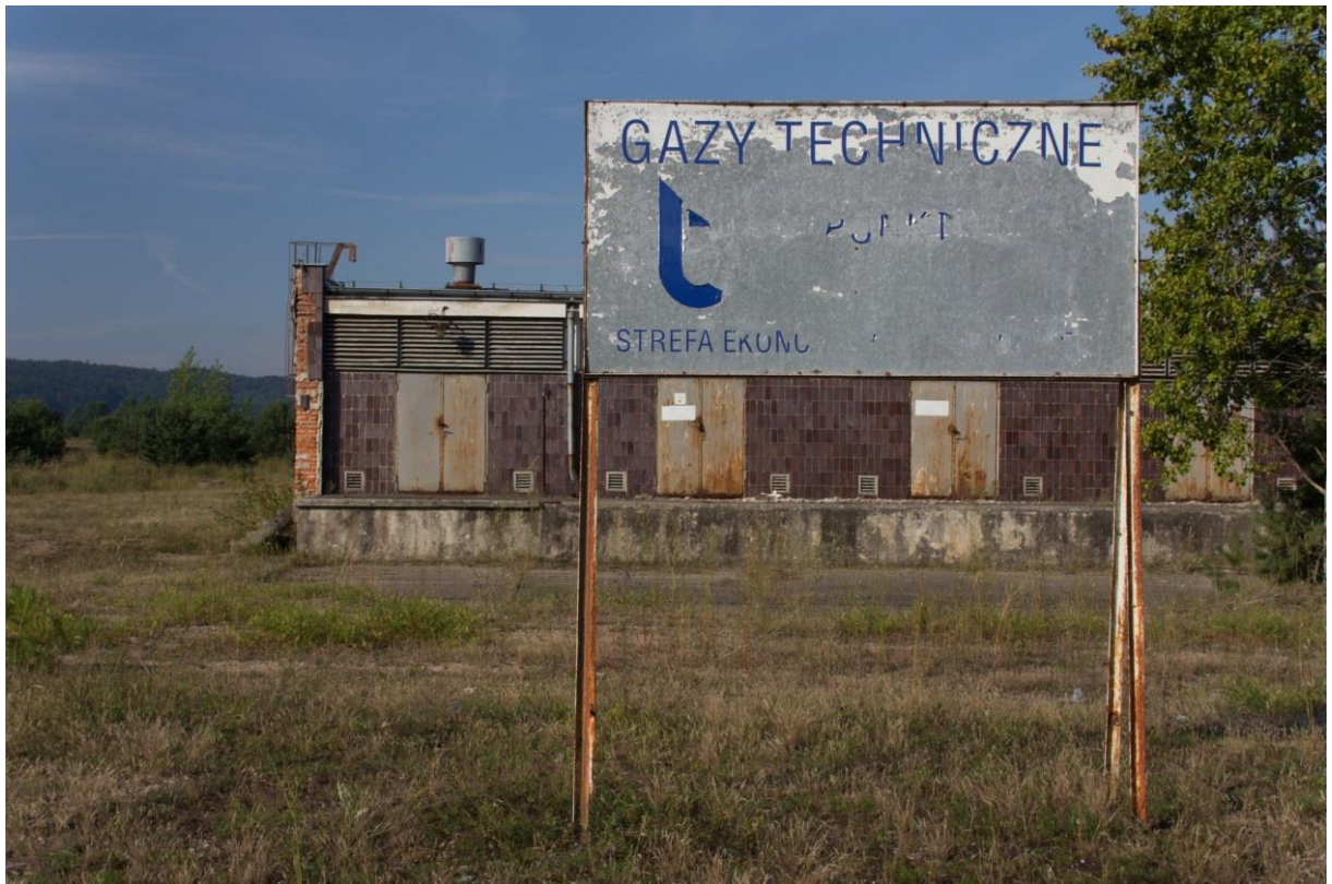
Figure 4.12 (marked 'D' in figure 4.1) As above (figure 4.11).
