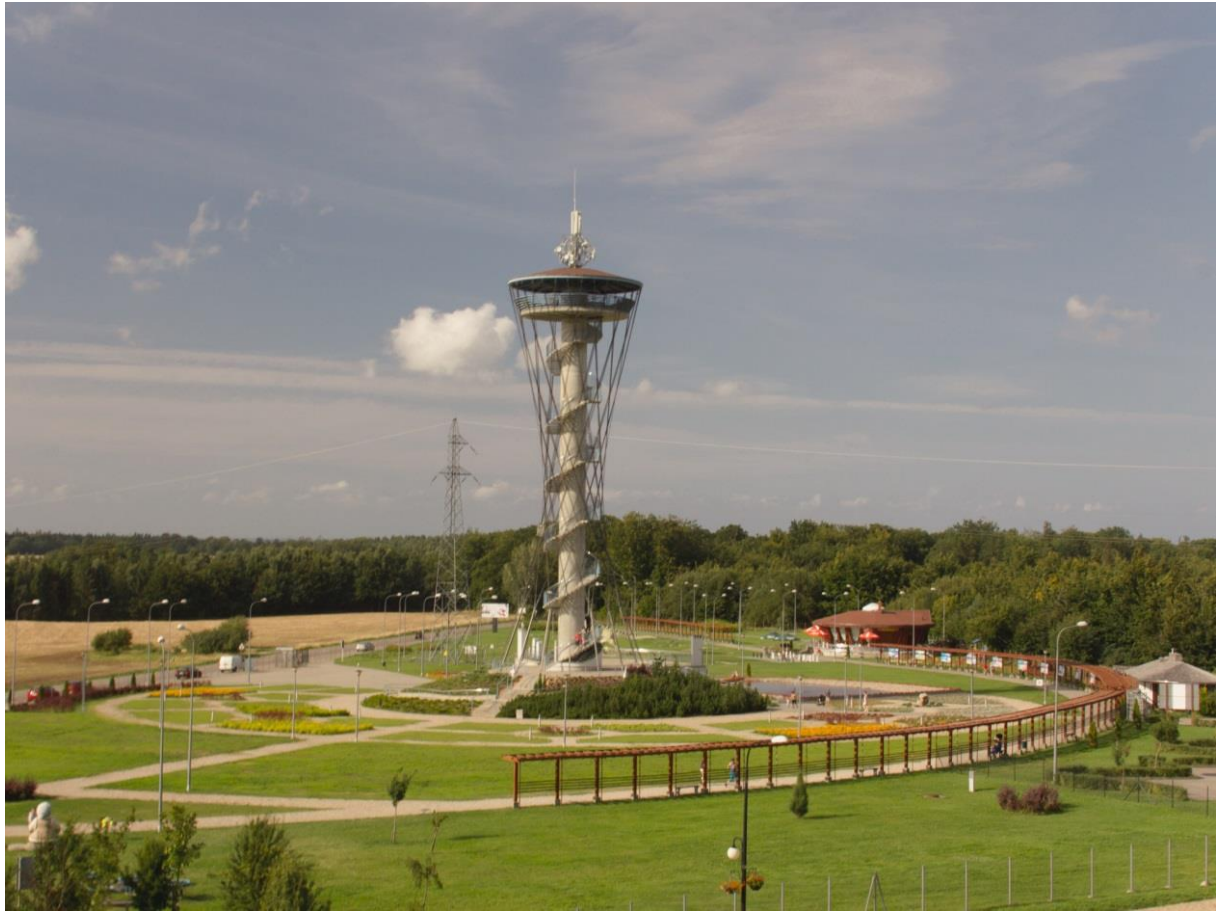
Figure 4.24 (marked ‘I’ in figure 4.1) The ‘Kashubian Eye’ as seen from the bank of the artificial reservoir (figure 4.22).
