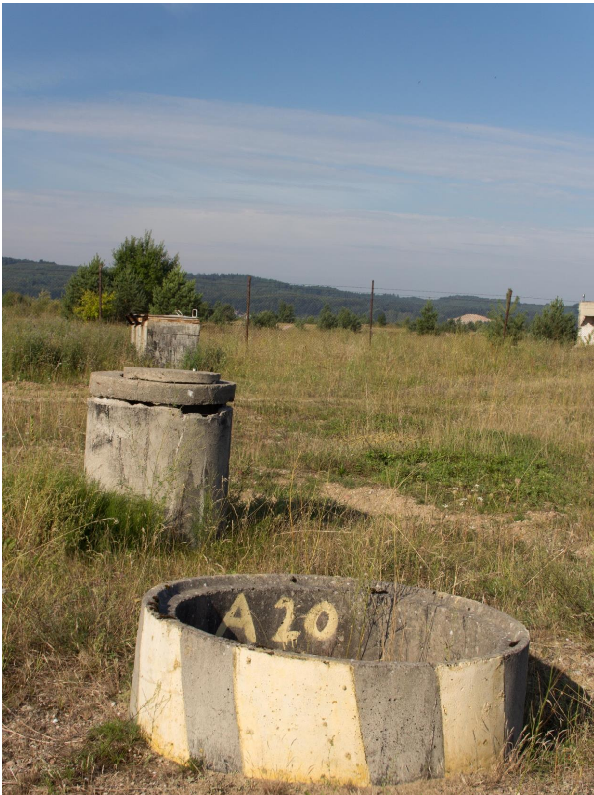
Figure 4.10 (marked 'C' in figure 4.1) The overgrown field in front of the reactor buildings. The land on which the ruins of Żarnowiec NPP sit formed, until 1982, farmland for the farming community of Kartoszyño.
