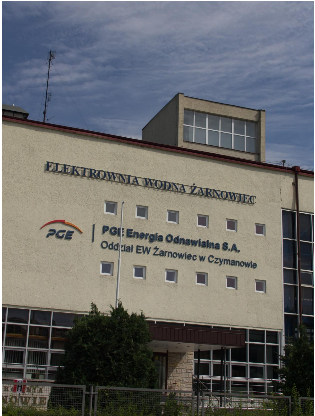
Figure 4.19 (marked 'H' in figure 4.1) Żarnowiec Hydroelectric, backing on to Lake Żarnowiec.
