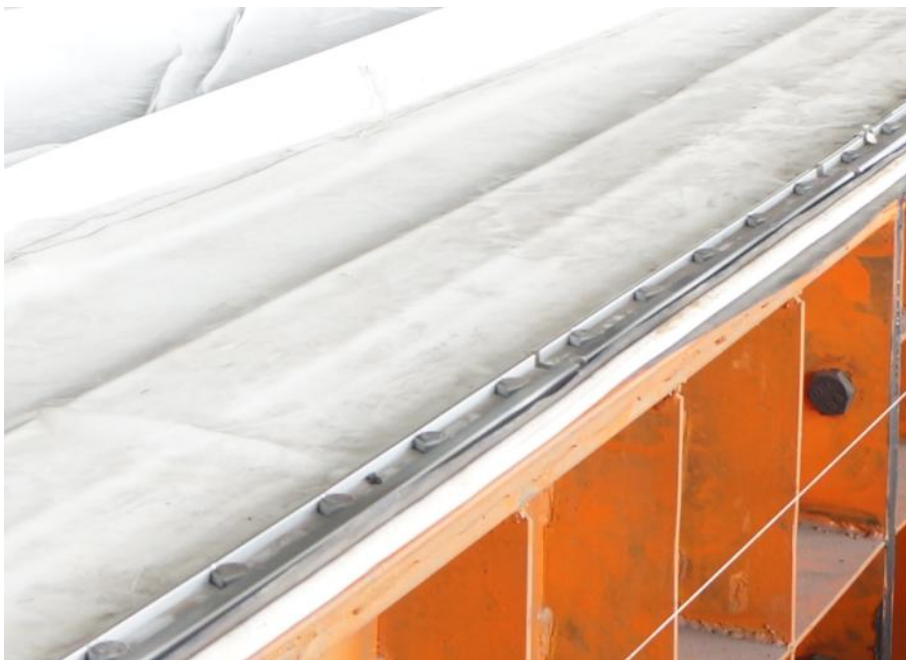
Figure 5-24: Screw fastening arrangement for the membrane seal
