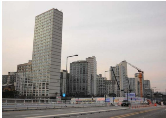
First Village Construction Site
