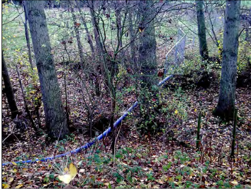
Figure 5-10: Photo D for Case Study 3, showing the unburied replacement water pipe
