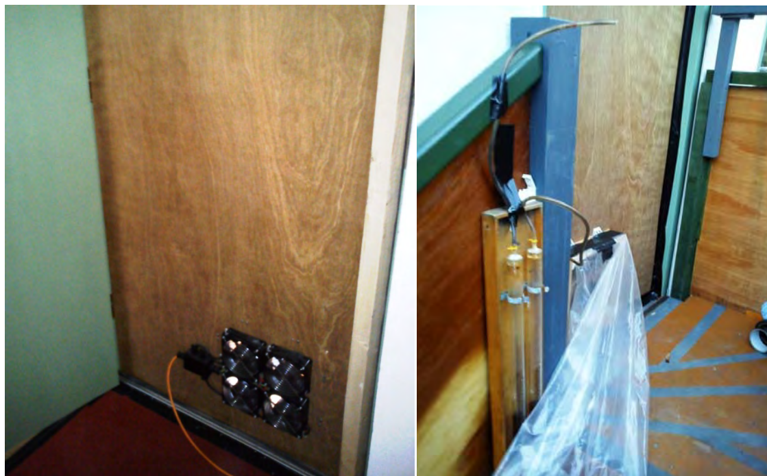
Figure 4-4: Axial fan fixed on portable timber door mounted at the door way and pressure gauge
