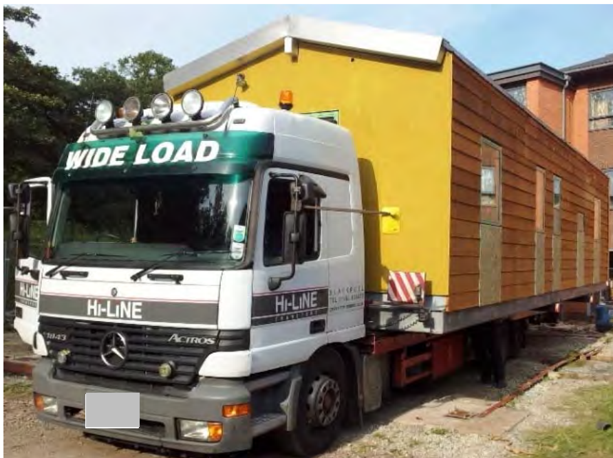
Figure 9-1: Extraction of EH unit from the construction site at the University of Birmingham, UK.
