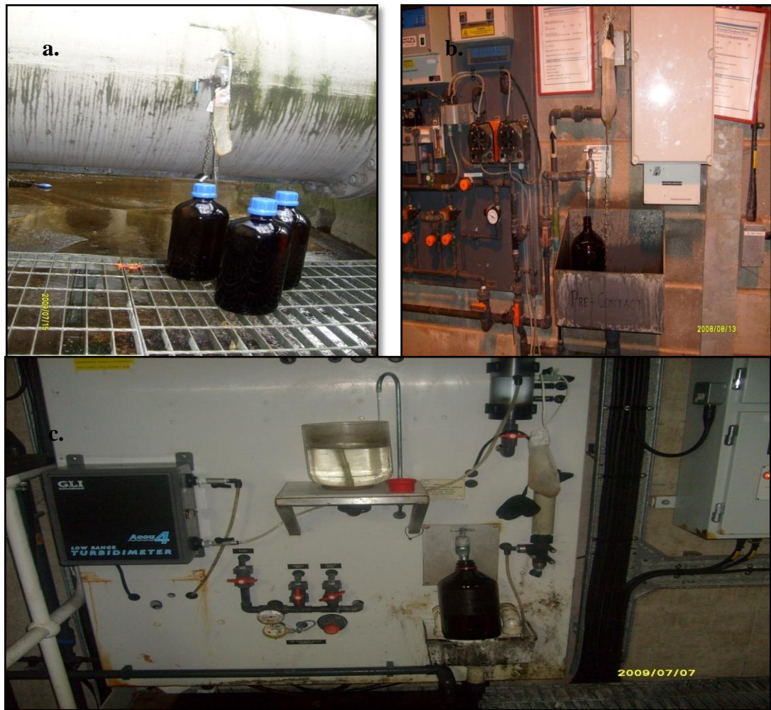
Figure 3-3: Photographs showing sample collection points of post-GAC water for a) Melbourne, b) Draycote, and c) Strensham WTWs, using brown 2.5l Winchester bottles.
