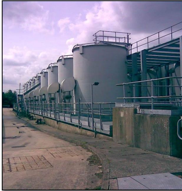
Figure 3-2: Photograph of drinking water post-GAC treatment units at Melbourne WTW
