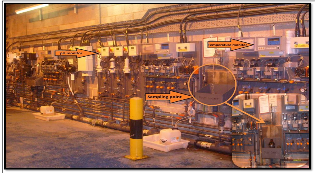
Figure 3-4: Photograph of the pH and Temperature monitors located at the post GAC water sampling point at Draycote WTW.
